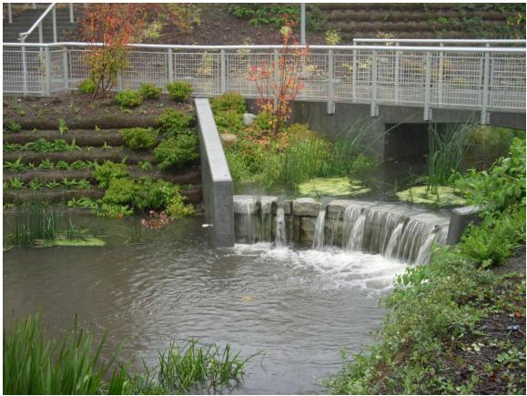
Figure 9 – Waterfall at Inlet to the Water Quality Channel
