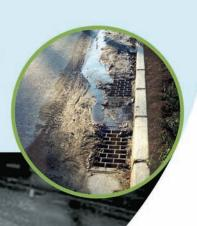
The sediment ponds slow down the flow of the stormwater and allow particles and pollutants to settle out. The water leaves the ponds through a small dam or weir. Weirs are located at the outlet of the sediment ponds and throughout the Channel to spread the flowing water across the wide Channel bottom. Although stormwater from 660 acres (500 football fields) joins the Channel here, runoff from some large storms will bypass in a pipe, protecting the Water Quality Channel from erosion.
