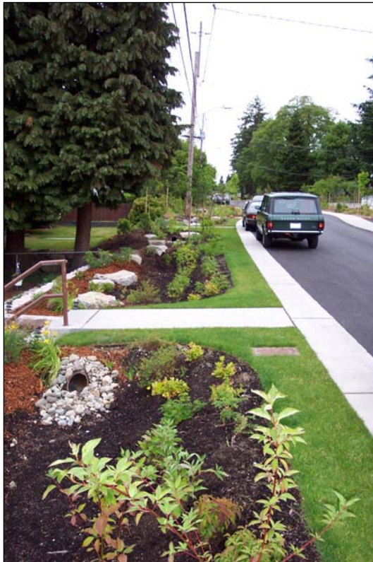
Figure 2. An attractively planted swale at Broadview Green Grid, Seattle, Washington.
