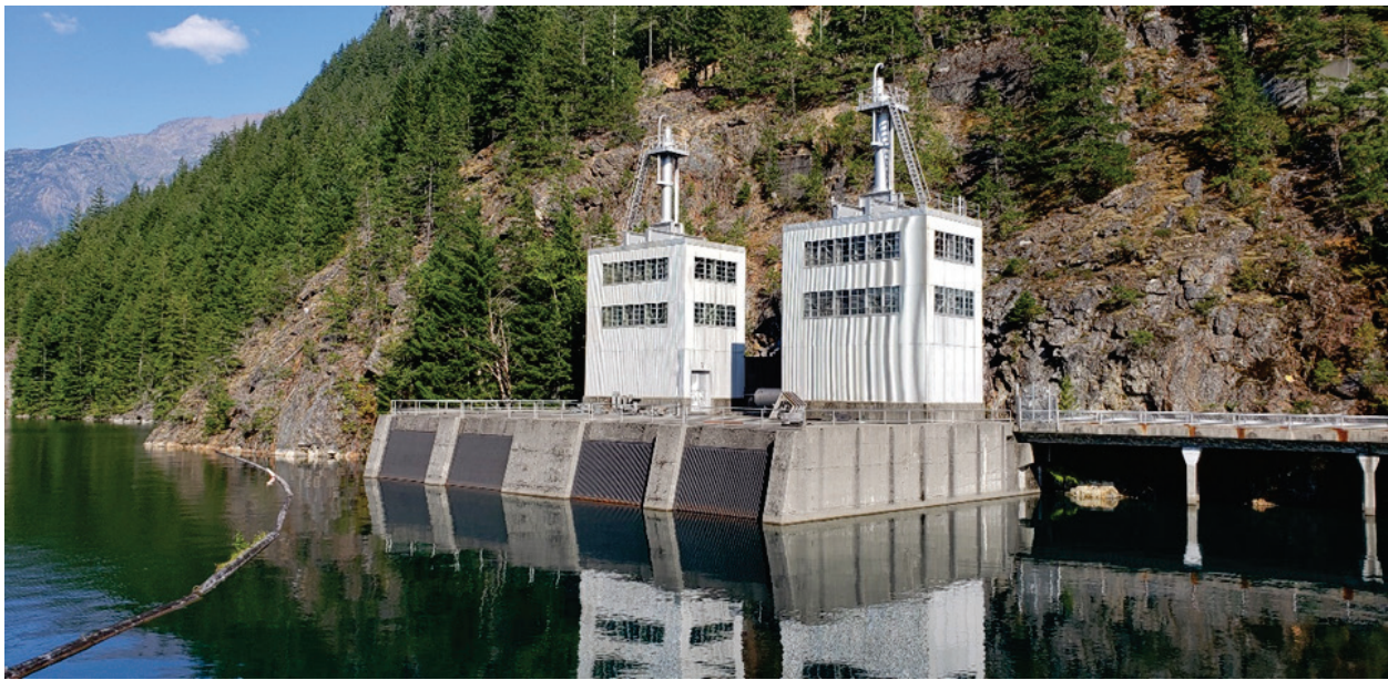
Figure 5.1-1. Ross power tunnel intake.
