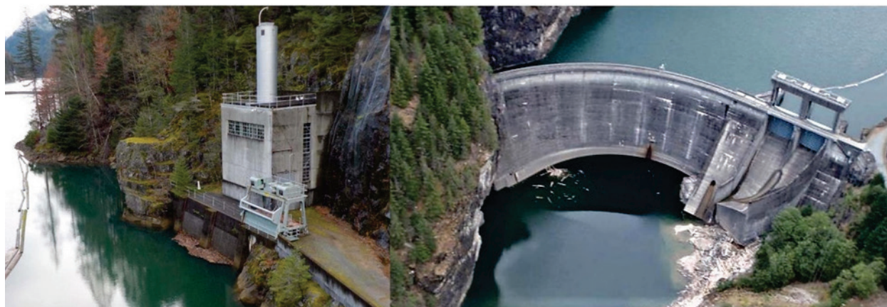
Figure 5.1-4. Gorge intake and dam with spillway.
