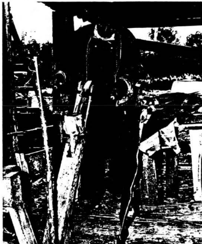
5. Custom Handsplitted shingles are still made the traditional way with a mallet and froe or ax. For these cypress shingles, a "bolt" section of log (photo A) the length of the shingle has been sawn and is ready to be split into wedge-shaped segments. Handsplitted shingles are fabricated with the ax or froe cutting the wood along the grain and separating, or riving, the shingle away from the remaining wedge. The rough surfaces are dressed on a shavinghorse using a draw-knife as shown above (photo B). Note the long wooden shingles covering the work shed in photo A. Photos: Al Honeycutt, North Carolina Division of Archives and History.
