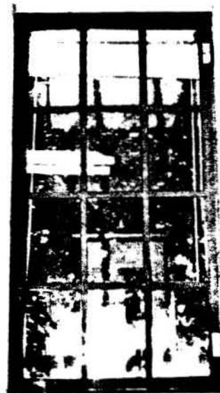
Fig. 6 d. View looking down towards the sill. The subframes appeared very rusted, but were in good condition once debris was vacuumed and surface rust was removed, in place, with chemical compounds. Where necessary, epoxy and steel filler was used to patch depressions in order to make the subframe serviceable again.
