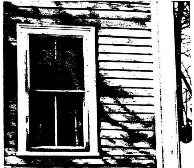
Figure 6. The addition of triple track storm windows, as shown here, greatly improves the thermal performance of existing window assemblies, with a minimal impact on the appearance of the building. (Photo: Baird Smith)
