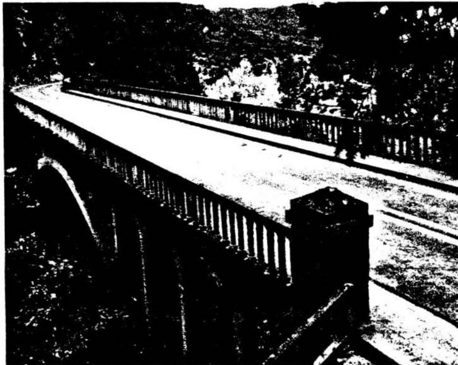
Fig. 15c. The new concrete spindles have been installed. This sensitive renovation reused the historic concrete cap railing and stone piers, as they were still in sound condition.
