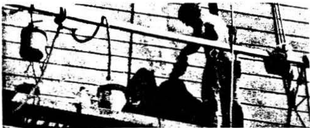
Fig. 13g. A soft brush is used to smooth the patch and to blend it with the adjacent historic concrete.
