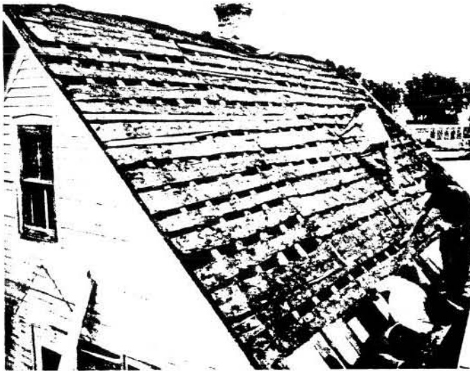
7. The reroofing of the circa 1856 Stovewood House in Decorah, Iowa, revealed the original open sheathing boards and pole rafters. Sawn cedar shingles were used as a replacement for the historic cedar shingles seen still in place at the ridge. A new starter course is being laid at the eaves. Photo: Norwegian-American Museum, Decorah, Iowa.
