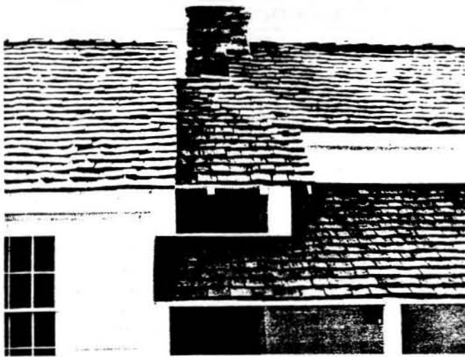
12. Inappropriately selected and installed wooden shingles can drastically alter the historic character of a building. This tavern historically was roofed with handsplit and dressed shingles of a relatively smooth appearance. In this case, a commercially available shake was used to effect a "rustic" appearance. Photo: National Park Service.
