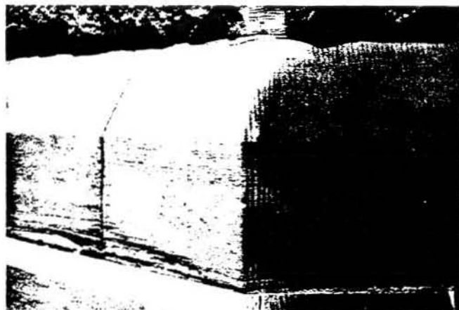
Abrasive Cleaning of Toolled Granite. Even this carefully controlled "wet grit" blasting has erased vertical tooling marks in the cut granite blocks on the left. Not only has the tooling been destroyed, but the damaged stone surface is now more susceptible to accelerated weathering.
