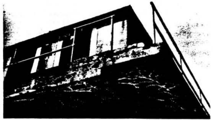
Fig. 7. Battery Commander's Station, Ft. Washington, Maryland (1904). This reinforced concrete tower with a cantilevered balcony is showing serious deterioration. Water has penetrated the slab, causing freeze-thaw spalling around the posts and corrosion of the reinforcing bars. This internal corrosion is causing expansion inside the slab and creating major horizontal cracks in the concrete. Under the balcony can be seen the network of hardened white calcified deposits, which have exuded through cracks in the concrete as a result of alkali-aggregate reaction. Photo: Lee H. Nelson, FAIA.
