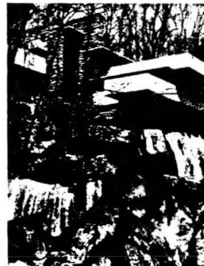
Fig. 5. "Fallingwater," near Mill Run, Pennsylvania (1936-37). This dramatic reinforced concrete residence by Frank Lloyd Wright is anchored into bedrock on the hillside and cantilevered over the stream. The great tensile strength of reinforced concrete made this type of construction possible. Photo: Paul Mayen.
