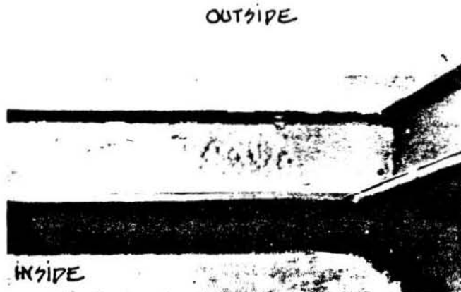
Fig. 6 e. View looking down towards the sill. The cleaned frame was reset in the window opening. The frame was screwed to the refurbished subframe at the jamb and the head only. The screw holes at the sill, which had been the cause of much of the earlier rusting, were infilled. Vinyl weatherstripping was added to the frame.
