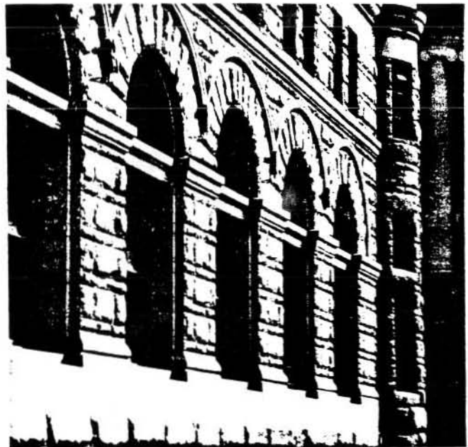
Figure 4. Heavy masonry walls in office buildings dramatically reduce the need for summer cooling because the thermal inertia (M factor) of the massive wall increases its thermal resistance (R factor), thus delaying the heat transfer into the building until late afternoon when the office workers have gone home. (Photo: Baird Smith)
