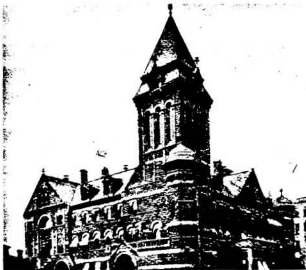
Figure 1. This 1891 Courthouse and Post Office in Rochester, New York, has built-in energy conserving features such as, heavy masonry walls, operable windows, an interior skylighted atrium which provides light and ventilation, and roof-top ventilators which keep the building cooler in the summer. Also note the presence of awnings in this old photograph.
