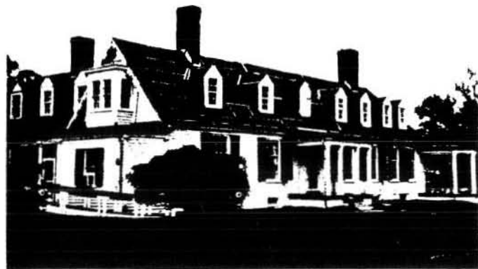
A. The later non-historic shingles were removed from Appomattox Manor (circa 1840 with later additions) and roofing paper was installed for temporary protection during the re-shingling.
