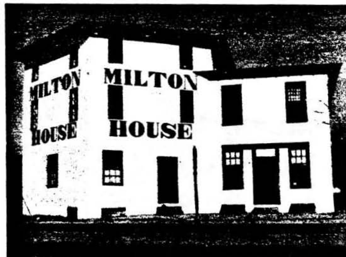
Fig. 1. Milton House, Milton, Wisconsin (1844). An early example of gravel wall construction with 12- to 15-inch thick monolithic concrete walls coated on the exterior with stucco. Photo: William B. Coney.
