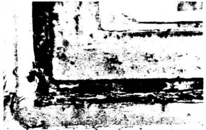
Fig. 6 b. View from the exterior showing the deteriorated condition of the lower corner of a window prior to repair. While the sash was in relatively good condition, the frame behind was rusted to the point of inhibiting operation.
