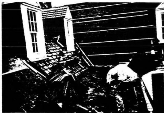
C. The replacement shingles (see specifications above), matched the historic shingles and were of such high quality that little hand dressing was needed at the site. The building paper, a temporary protection, was removed as the shingles were installed on the sheathing boards.
