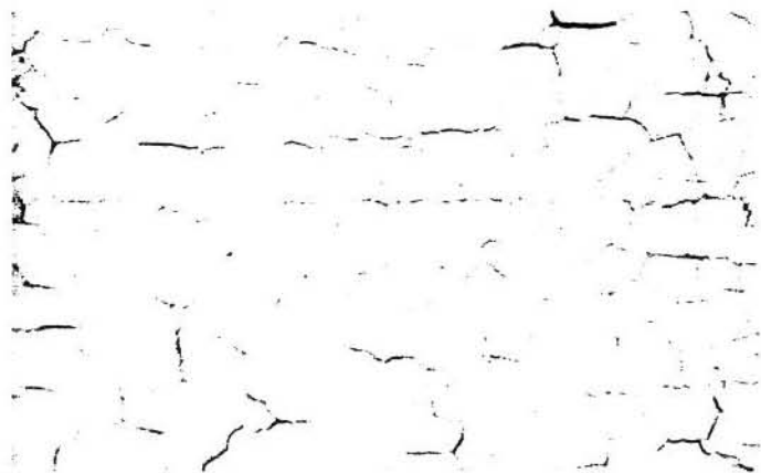
Fig. 5 Crazing—or surface cracking—is an exterior surface condition which can be successfully treated by sanding and painting. Photo: Courtesy, National Decorating Products Association.
