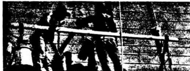
Fig. 13f. Workmen are applying patching concrete and using a trowel to form ridges to match the appearance of the historic concrete ridges that were originally created by the form boards.
