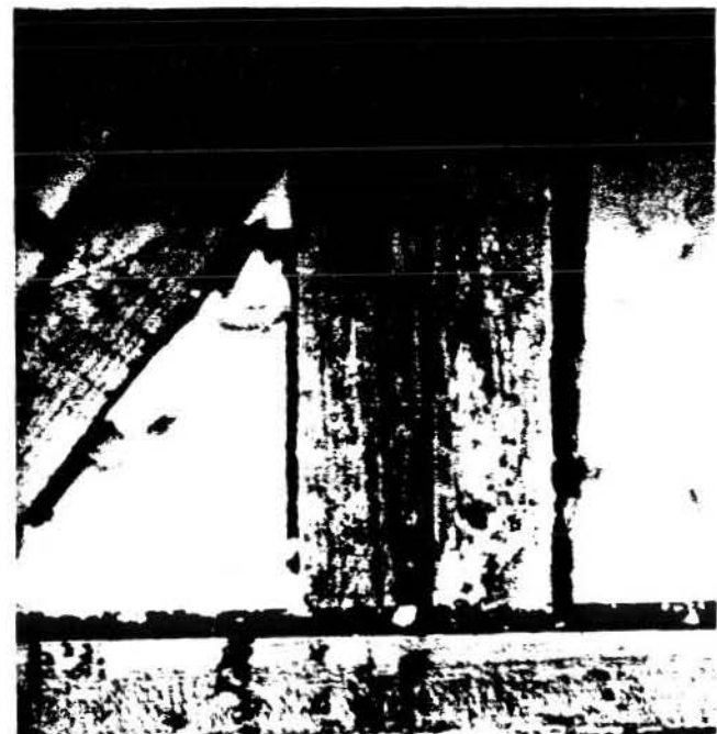
Figure 8. The white material seen between the wooden wall studs is urea-formaldehyde foam. It is injected into the wall cavity wet, and as it cures, large quantities of moisture are given off creating the potential for serious deterioration of adjacent materials and may cause paint to blister on interior and exterior wall surfaces. Additionally, foam can shrink as much as that shown here (about 7% by volume), thus reducing the predicted insulating performance. Until some of the technical problems are corrected, its use is not recommended in historic structures. (Photo: Baird Smith)
