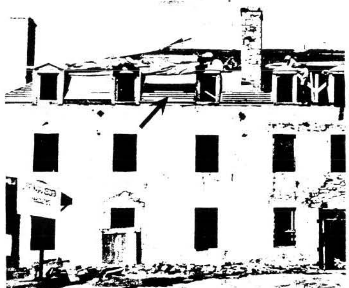
9. This 1927 view of the reroofing of the French Castle at Old Fort Niagara, N.Y., shows the wooden sleepers being laid (see arrow) over solid sheathing in order to raise the shingles up slightly to allow under-shingle ventilation. Note that the horizontal strips are not continuous to allow airflow and trapped moisture to drain away. This cedar roof has lasted for over 60 years in a harsh moist environment. Photo: Old Fort Niagara, Assoc. Inc.
