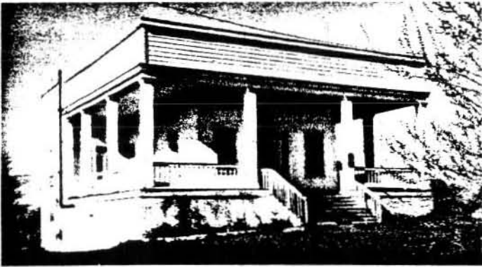
Fig. 2. Sebastopol House, Seguin, Texas (1856). This Greek Revival dwelling is one of the few remaining poured-in-place concrete structures in this Texas town noted for its construction of over 90 concrete buildings in the mid-nineteenth century. The high parapets surrounding the flat roof were lined and served as a water reservoir to cool the house. Photo: Texas Historical Commission.
