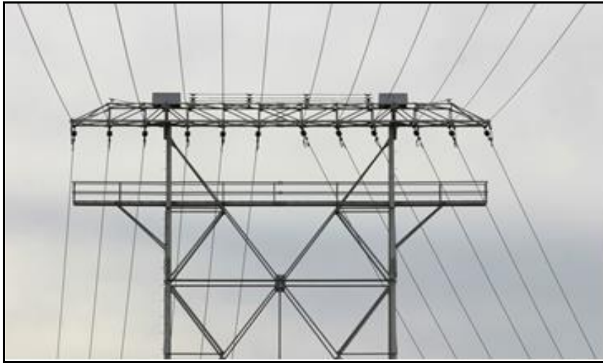
Figure 6.4 Tent covers on H-frame transmission towers
