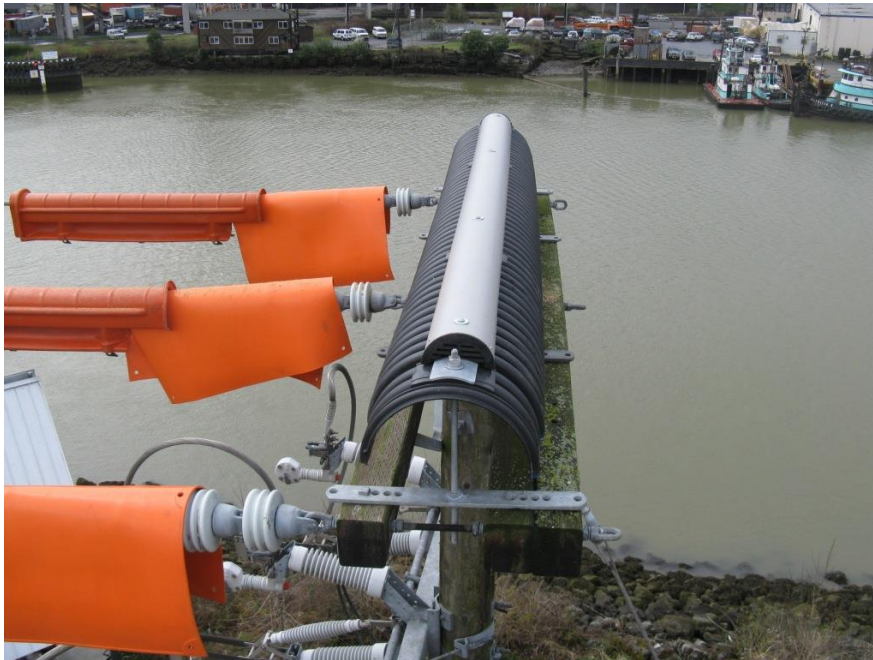
Figure 6.3 Osprey nest excluder and insulated conductor cover
