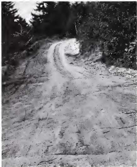
Figure 17.—Roads, during the construction phase, and if left unsurfaced after construction, are a major source of drainage system sedimentation.
