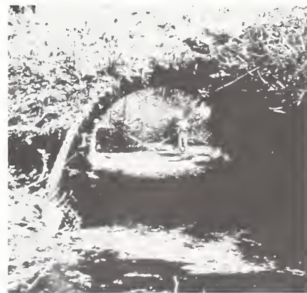
Figure 11.—Open bottom culverts and bridges make the best road crossing structures on salmonid streams.
