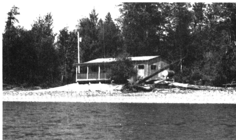
A fishing cabin built on uplatted private property above Rockport. A thick concrete foundation secures this cabin against high water. The structure has galvanized metal siding.
