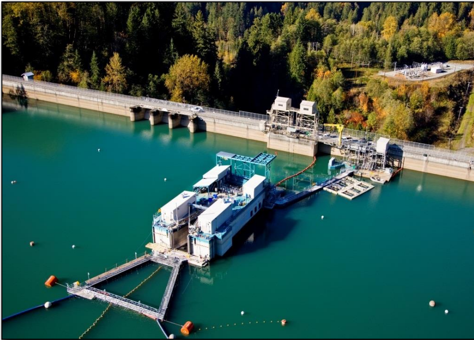
Floating Surface Collector (FSC) Upper Baker Dam, WA (photo by PSE)
