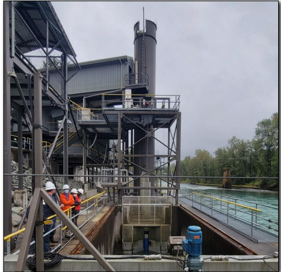
Fish lock at the trap and transport facility on Lower Baker River
