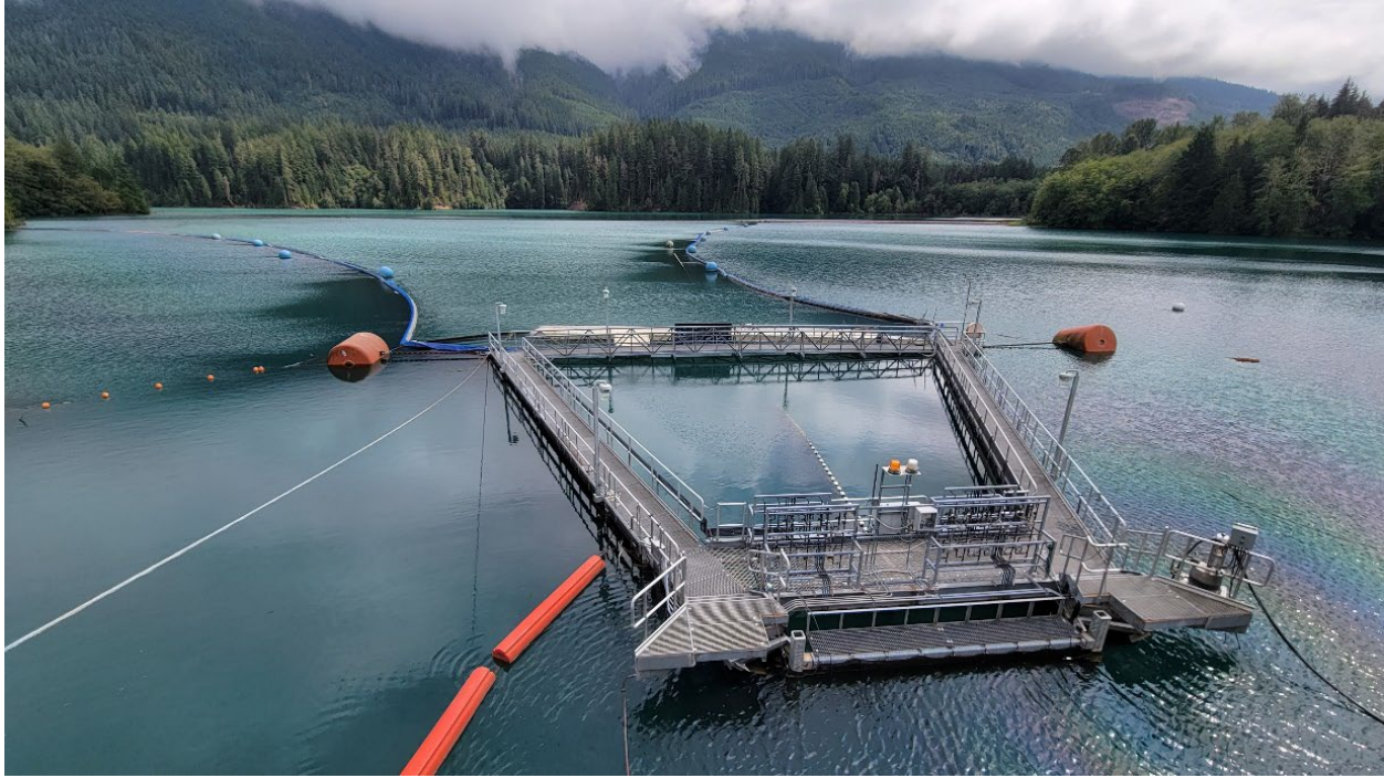
Figure 7.2-19. Net transition structure for Upper Baker FSC on Baker Lake upstream of Upper Baker Dam operated by PSE.
