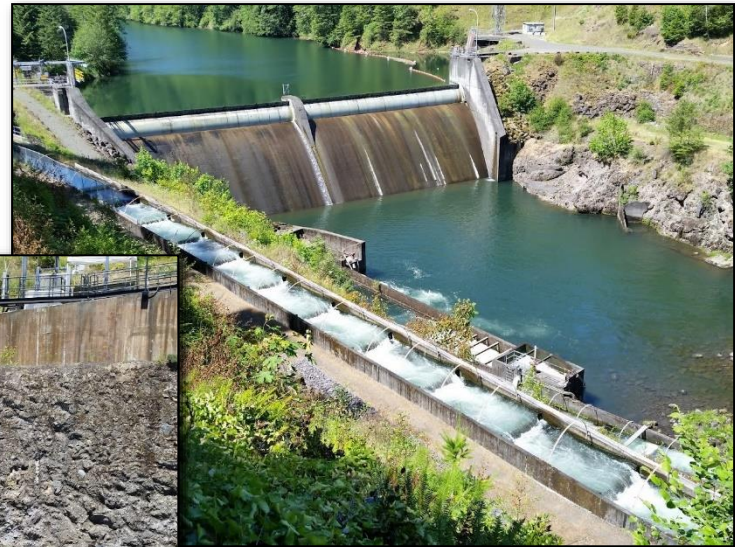
2.1 mile long half, Ice-Harbor baffle (pool, weir, and orifice) fish ladder at the Faraday Diversion Dam and North Fork Dam.
