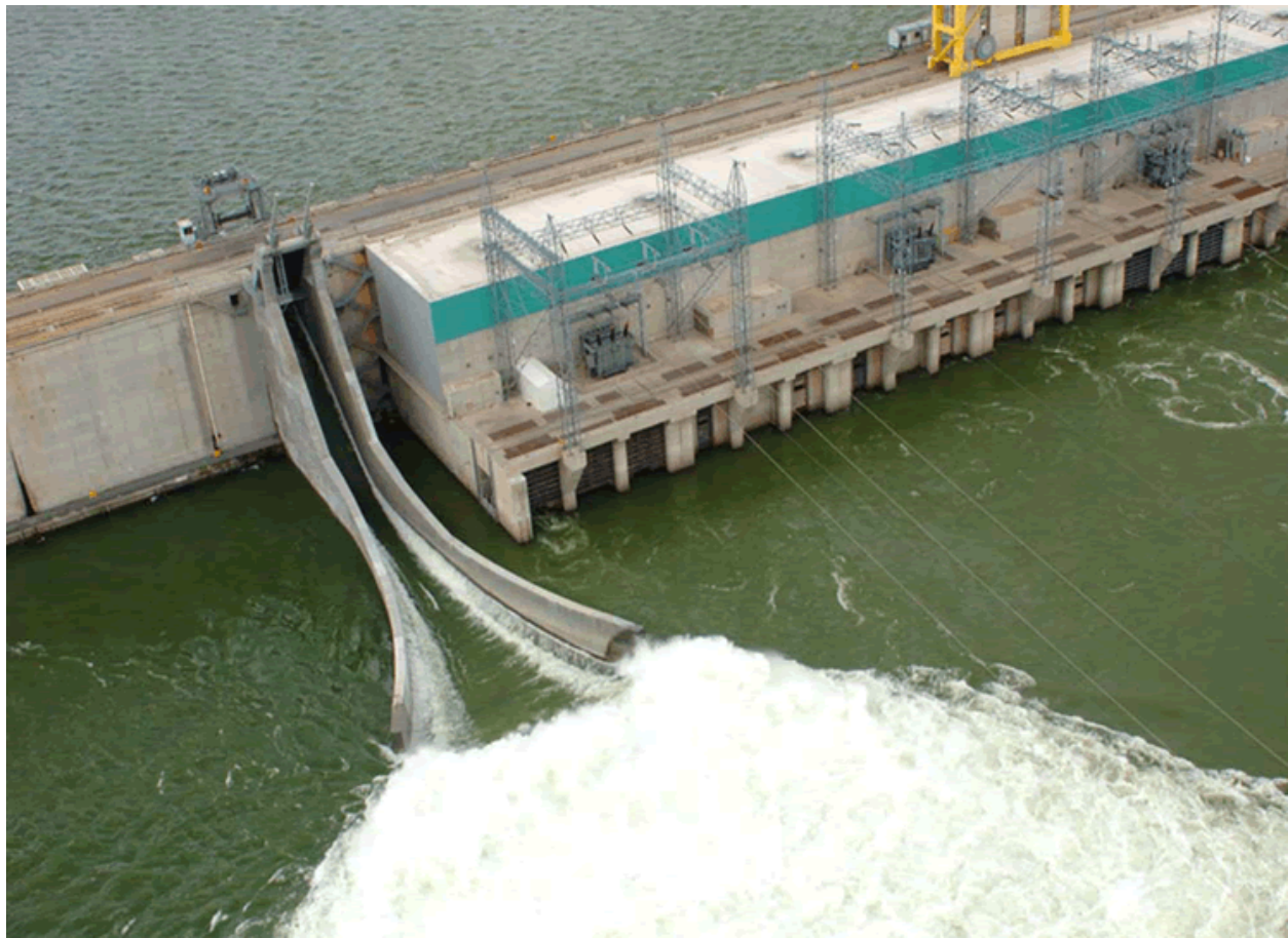
Figure 7.2-25. Example spillway weir and fish bypass flume at Wanapum Dam, Columbia River, Washington.
