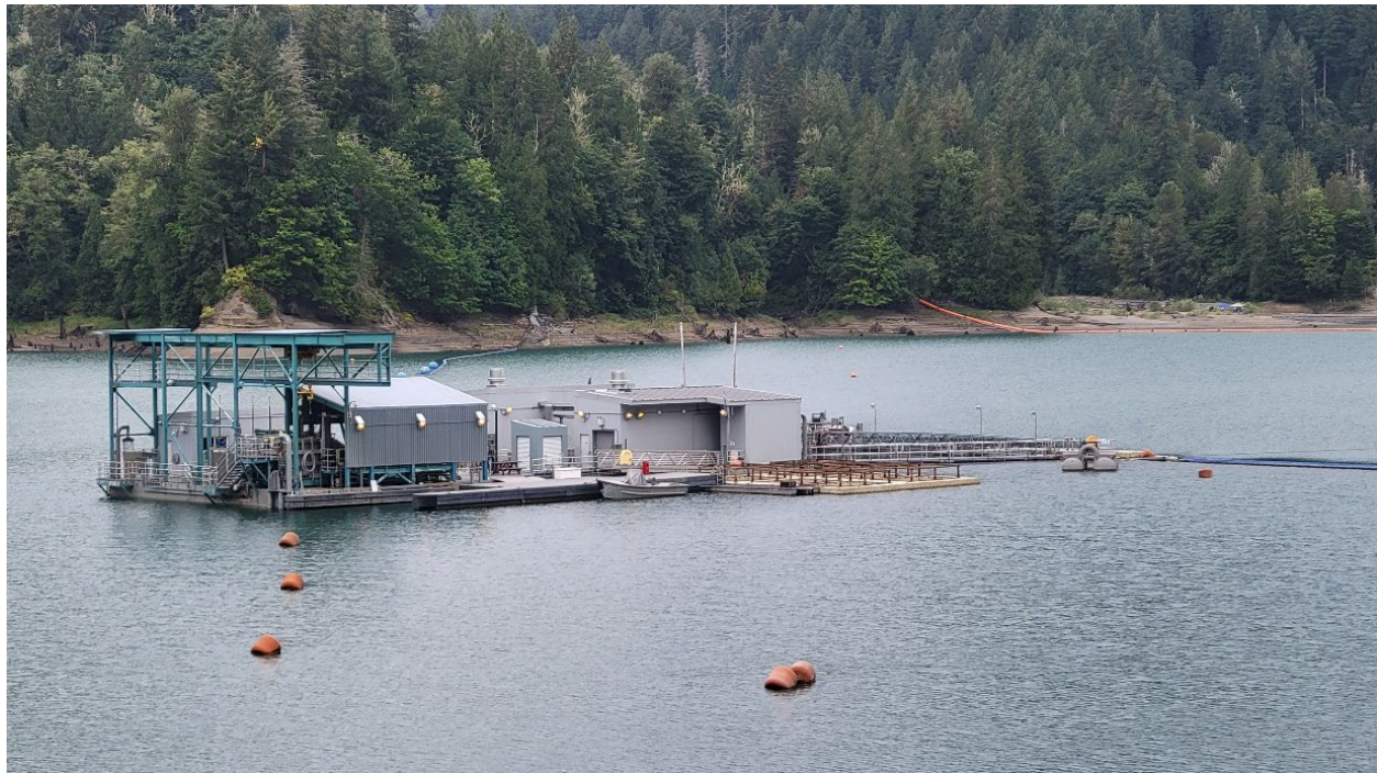
Figure 7.2-18. FSC on Lake Shannon upstream of Lower Baker Dam operated by PSE.
