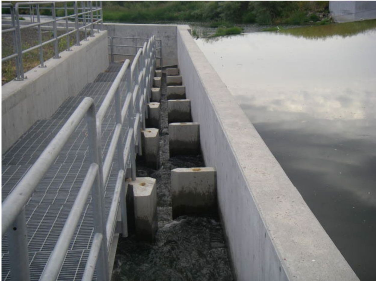
Figure 7.2-7. Crooked River central vertical slot fishway near Prineville, Oregon. Source: ODFW 2021.
