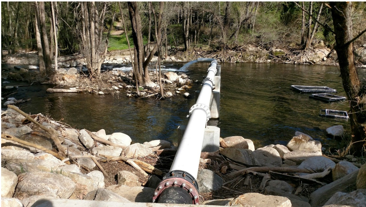
Figure 7.2-26. Example of 1,100-foot-long juvenile fish bypass and outfall at Los Padres Dam, Carmel River, California.
