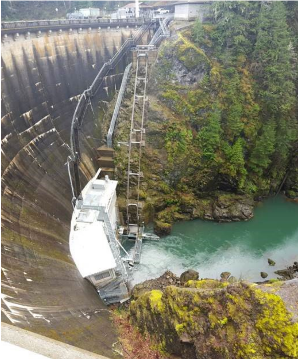
Figure 7.2-9. Skokomish Dam No. 2 Adult Collection Facility fish lift.
