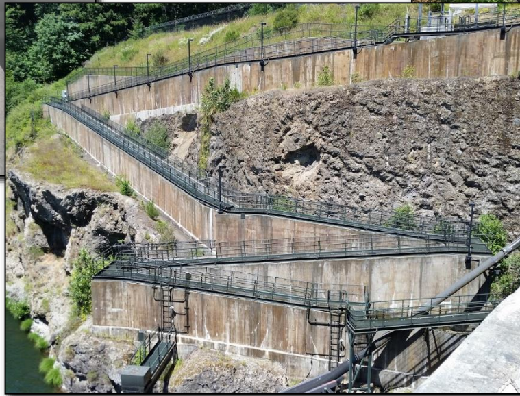
Half Ice-Harbor baffle (pool, weir, and orifice) fish ladder at River Mill Dam.
