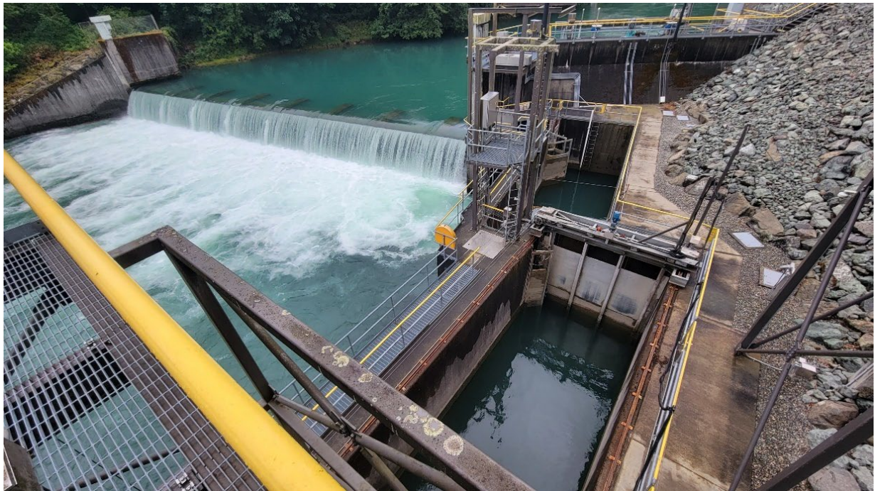
Figure 7.2-2. Lower Baker River adult trap and transport facility: barrier dam and collection/crowding gallery.
