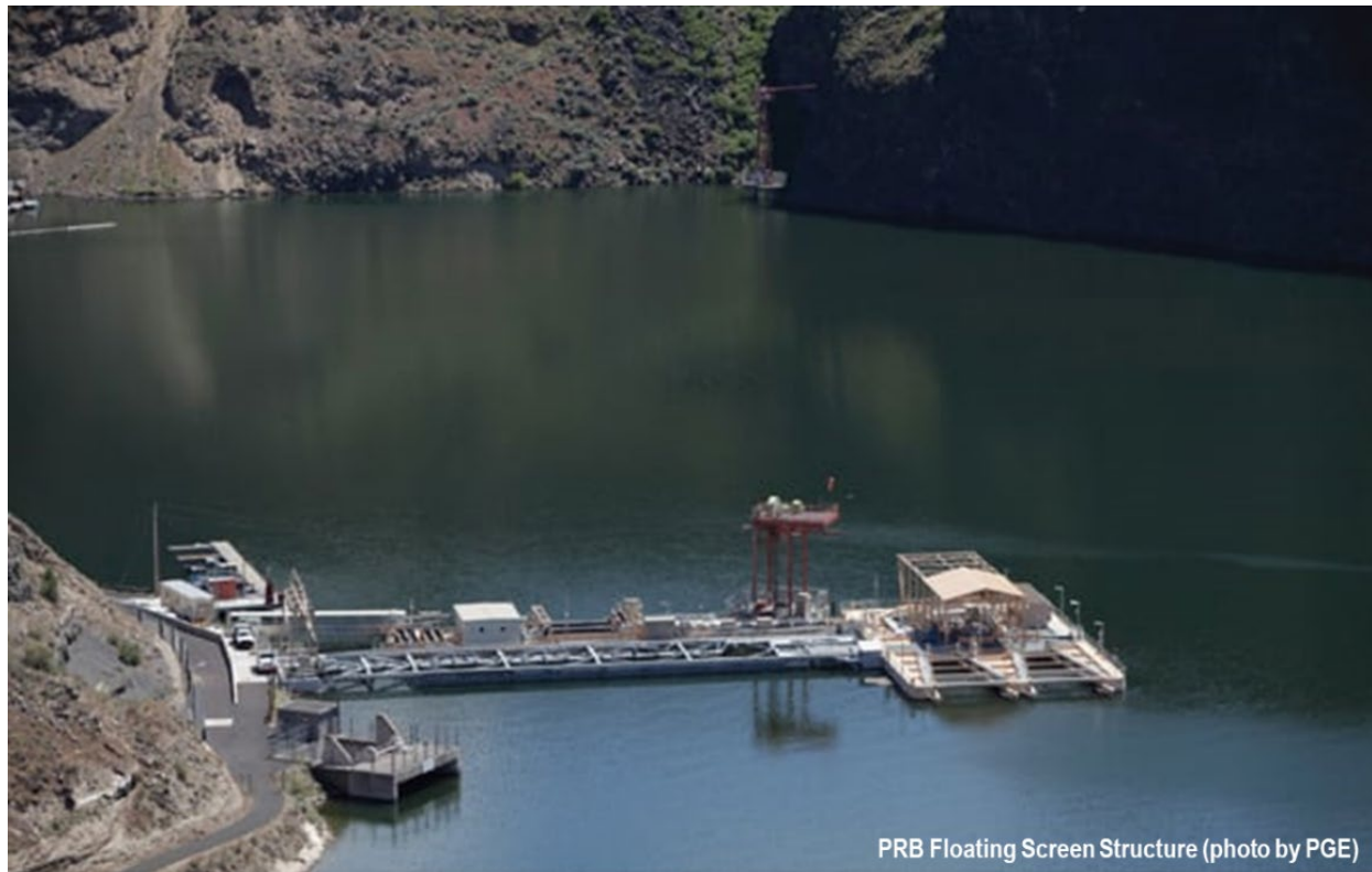
Figure 7.2-21. Photo of FSS on Deschutes River in Oregon, upstream of Pelton Round Butte Dam operated by PGE.
