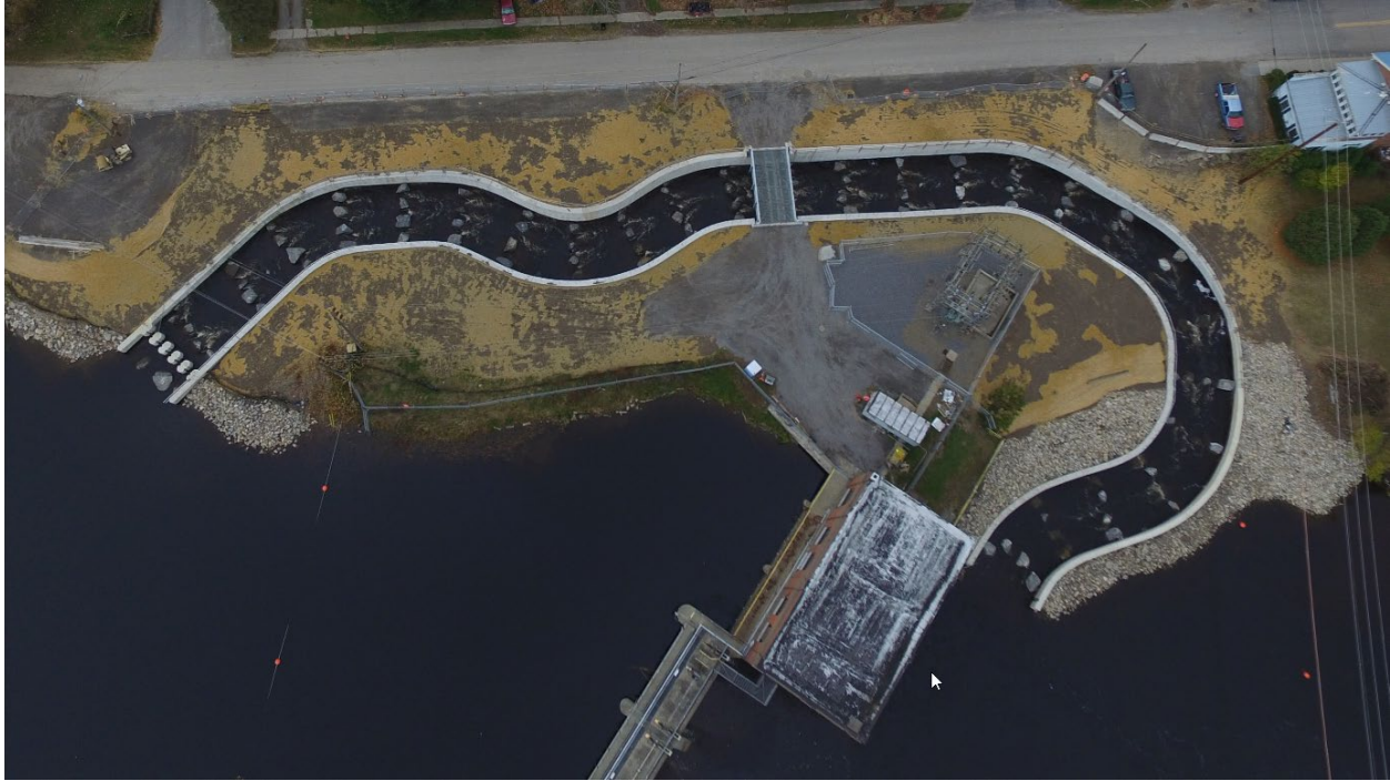
Figure 7.2-8. Heuvelton nature-like fishway on the Oswegatchie River in New York.
