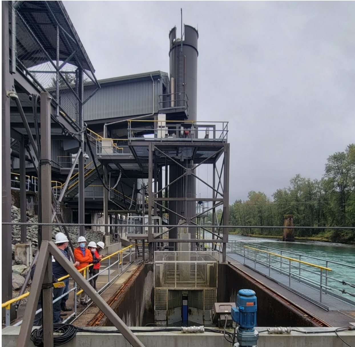
Figure 7.2-10. Fish lock at the trap and transport facility on Baker River operated by Puget Sound Energy.
