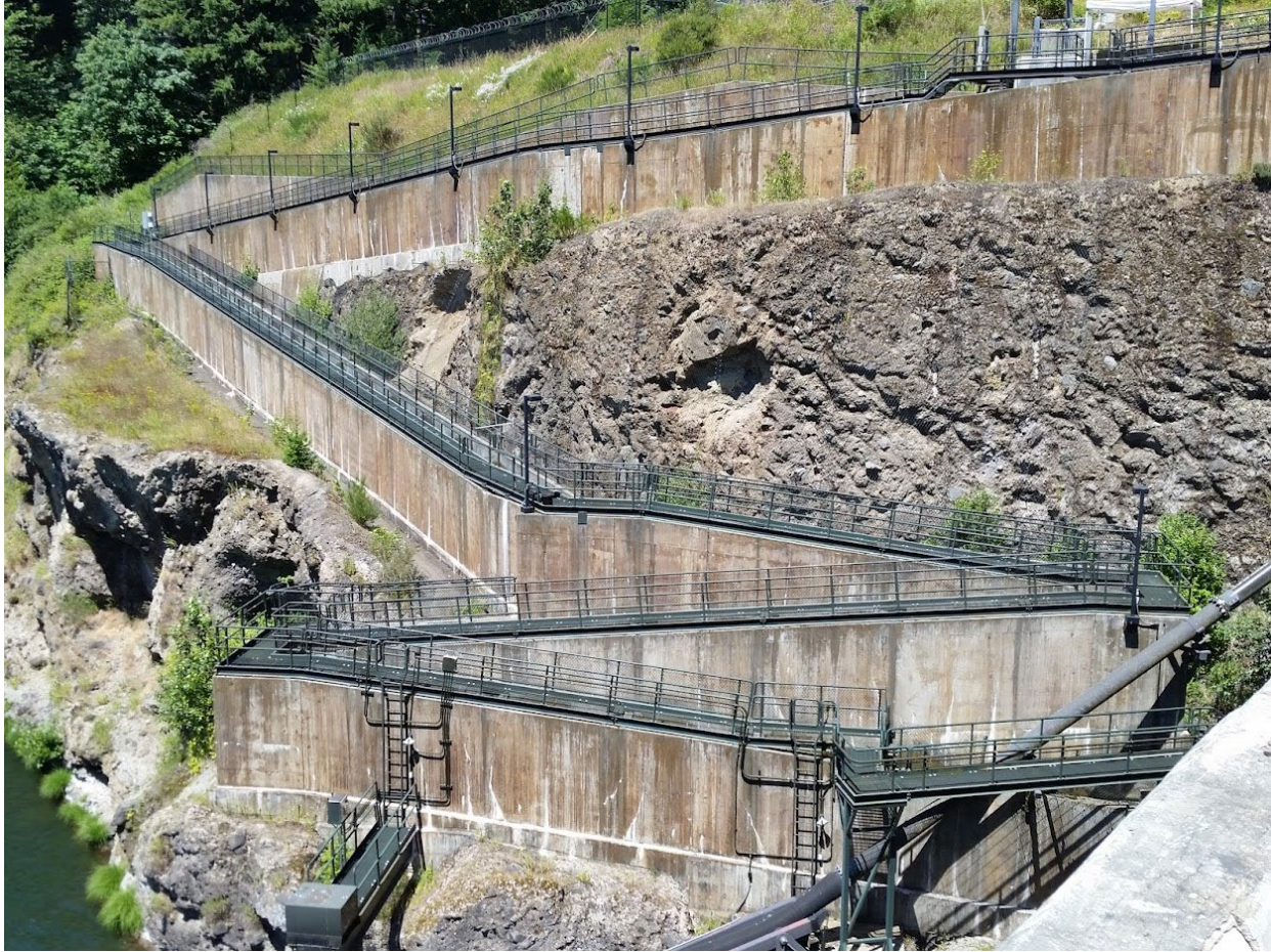
Figure 7.2-6. Half Ice-Harbor baffle (pool, weir, and orifice) fish ladder at River Mill Dam.
