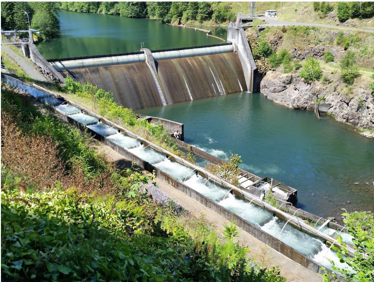
Figure 7.2-5. The 2.1-mile-long half, Ice-Harbor baffle (pool, weir, and orifice) fish ladder at the Faraday Diversion Dam and North Fork Dam.
