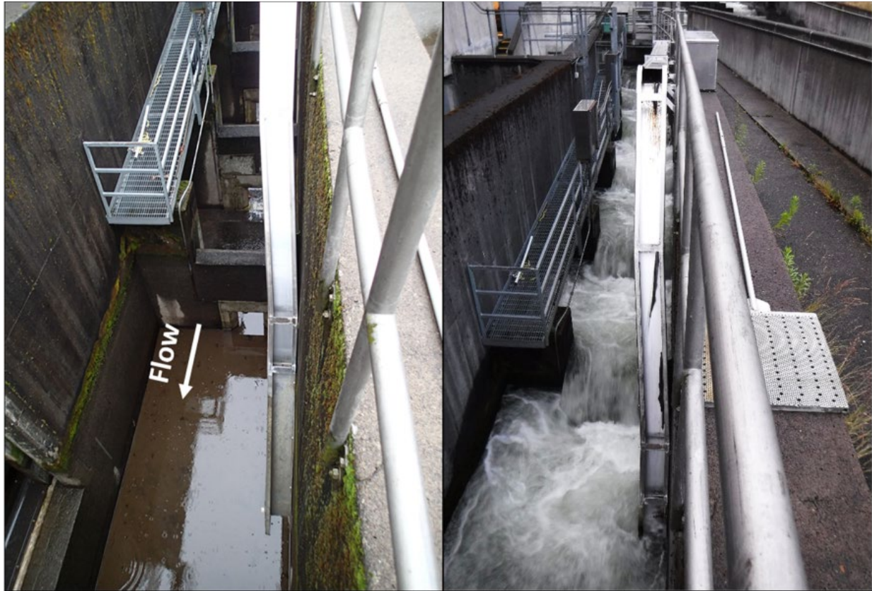
Figure 7.2-15. Bonneville Dam adult fish facility lamprey trap dewatered (left) and in operation (right). Source: Clabaugh et al. 2020.
