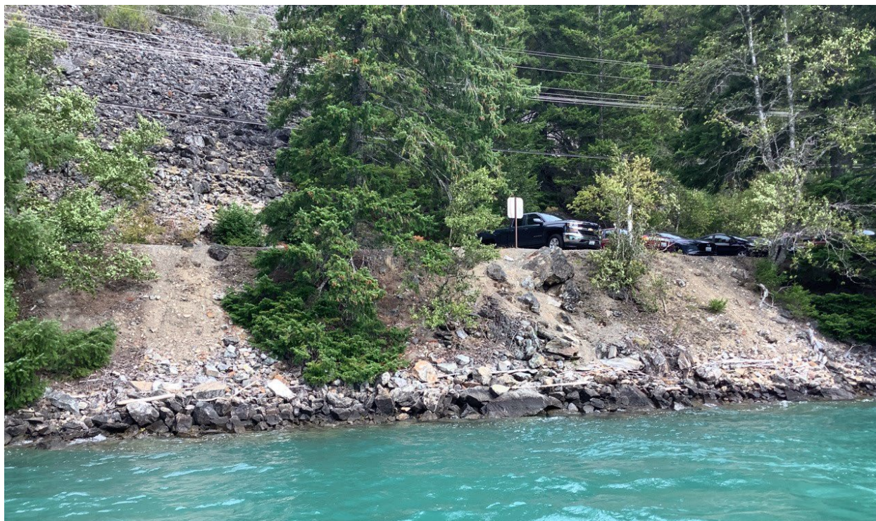
Figure 5.1-7. Erosion and rilling from road runoff observed at Project reservoirs.
