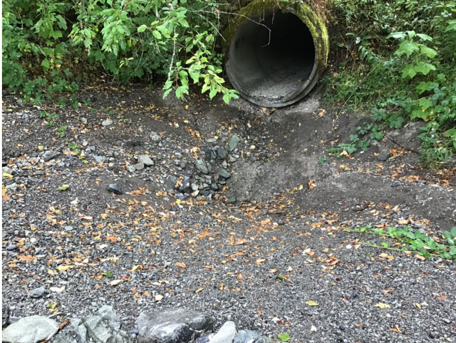
Figure G-57. Looking upstream at the outlet of the PCC culvert beneath State Rt. 20 that acts as a total fish barrier (WDFW 2021) on Sutter Creek.
