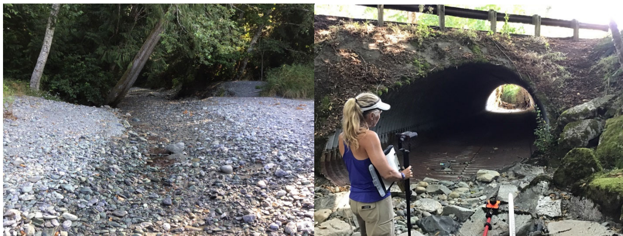
Figure G-44. Standing at mouth of Olsen Creek looking upstream (left). A surveyor stands at the downstream end of the squashed CMP beneath State Rt. 20 (right).
