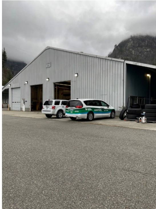
Figure 5.2-1. Gorge Switchyard and Maintenance Yard – typical wall packs (exterior lighting).
