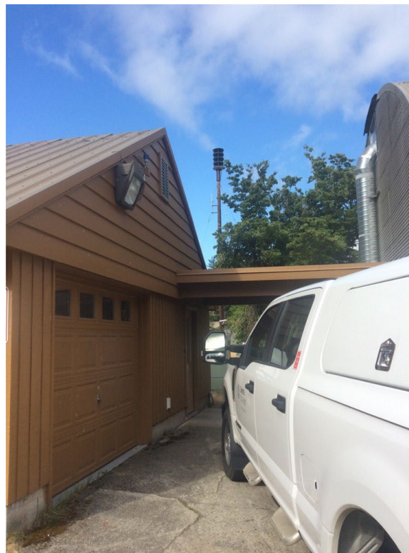
Figure 5.1-21. Newhalem administrative office garage driveway lighting – flood wall pack.
