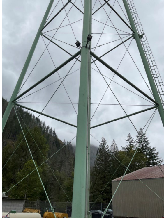
Figure 5.2-3. Gorge Switchyard and Maintenance Yard – typical exterior work area flood lighting.
