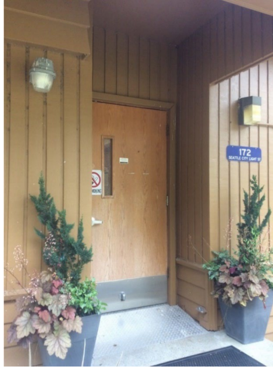
Figure 5.1-14. Newhalem administrative office entrance (typical pedestrian scale exterior wall pack luminaires).
