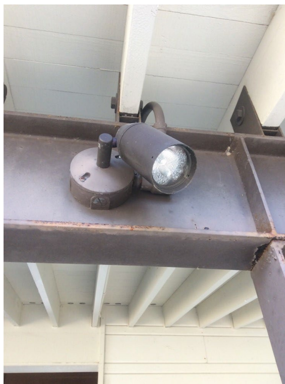
Figure 5.1-35. Newhalem Skagit Information Center lighting – typical adjustable flood lighting.
