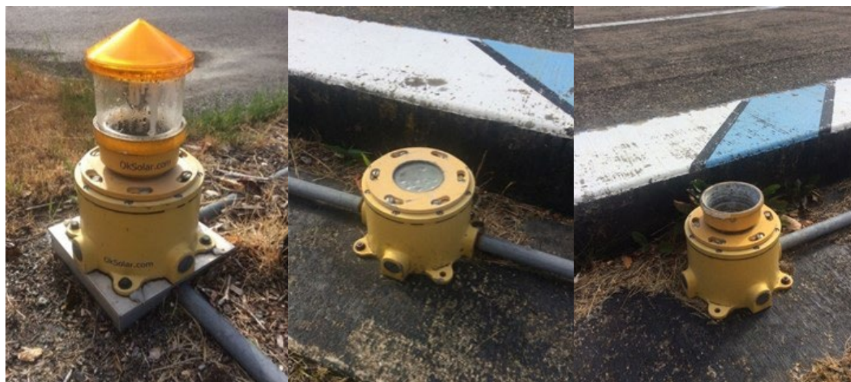
Figure 5.1-8. Newhalem helipad lighting (close-up views).
