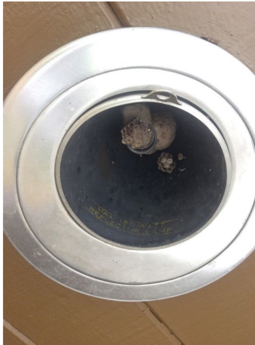
Figure 5.1-44. Newhalem – Currier Hall – typical exterior lighting (many luminaires are missing sources or have been replaced by new adjacent luminaires).
