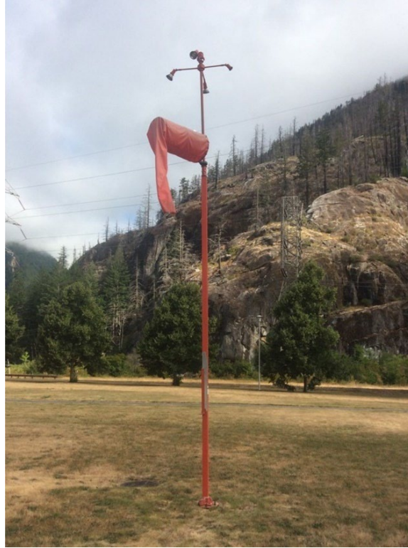
Figure 5.1-4. Newhalem helipad windsock flagpole lighting.
