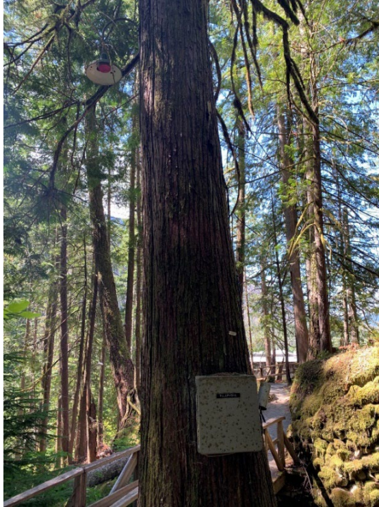
Figure 5.4-8. Ladder Creek Falls Trail and Garden original lighting – colored lamps, electrical equipment attached to tree trunks.
