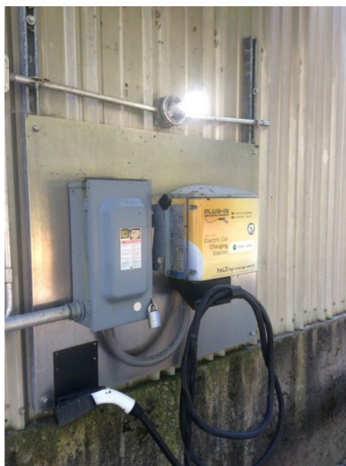
Figure 5.1-50. Gorge Switchyard and Maintenance Yard – City Light facility EV charging station (exterior lighting).
