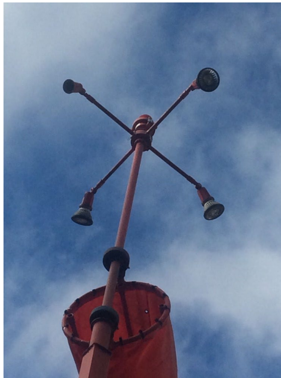
Figure 5.1-5. Newhalem helipad windsock flagpole lighting (close-up view).
