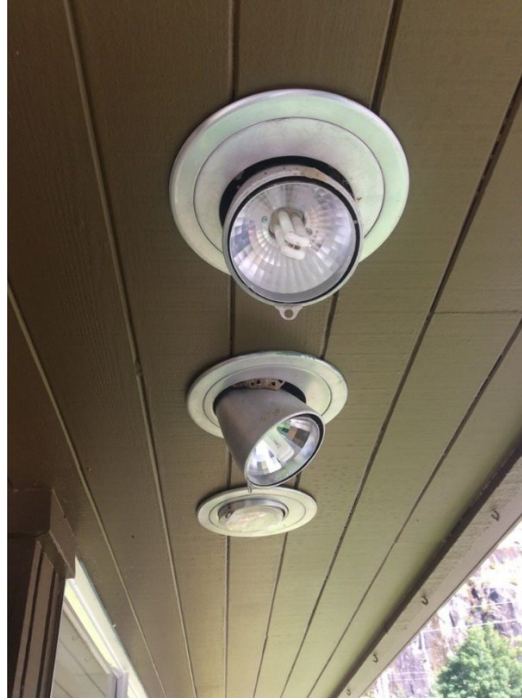
Figure 5.1-43. Newhalem – Currier Hall – typical exterior lighting (many luminaires are missing sources or have been replaced by new adjacent luminaires).
