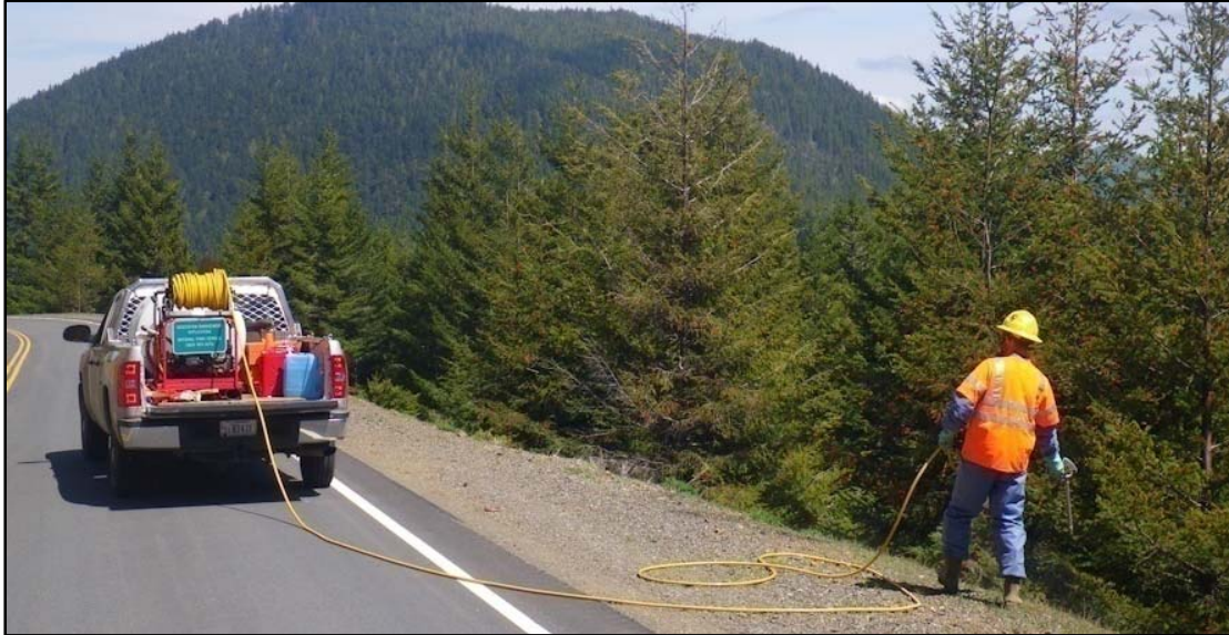
Figure 2-5. Roadside spot spraying
