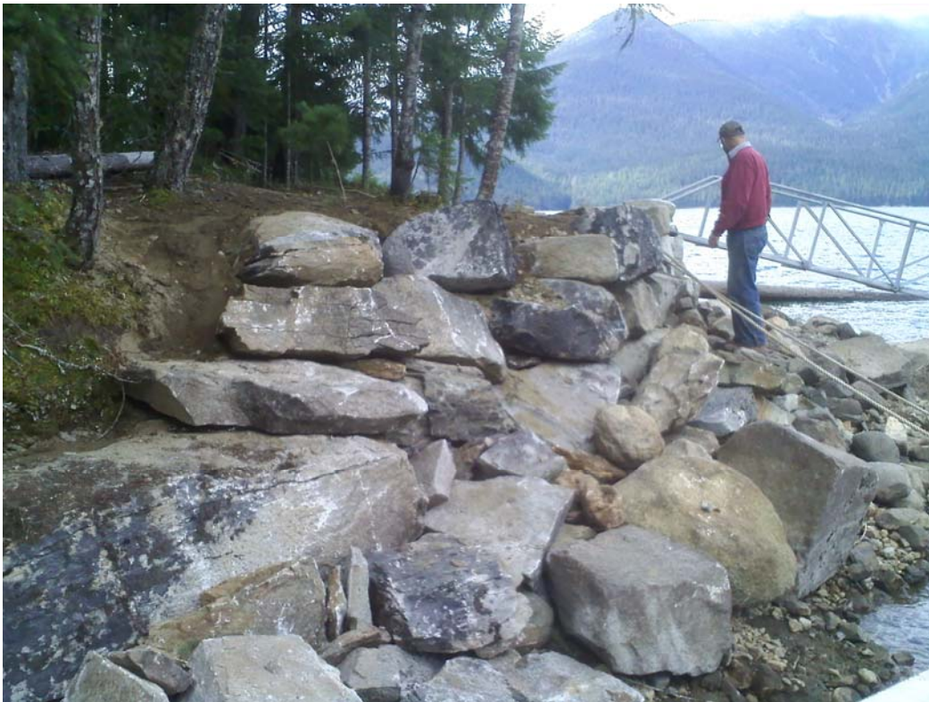
Photo 2: May Creek-after erosion control work (2009).
