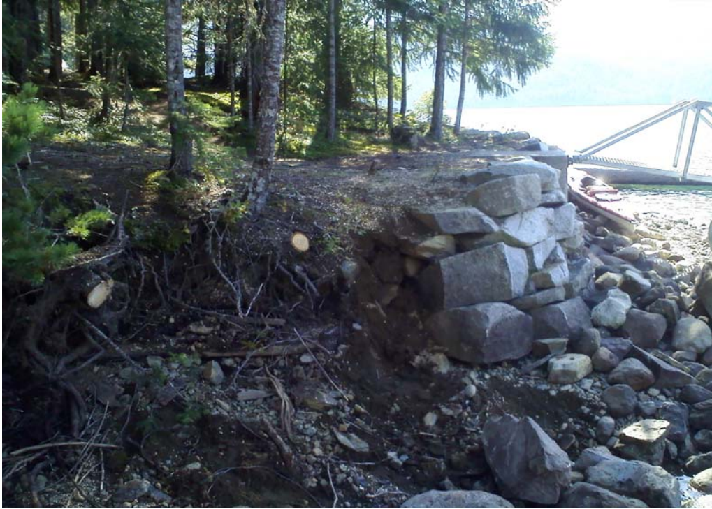
Photo 3: Crane places rock at Ten Mile Island site. (2009).
