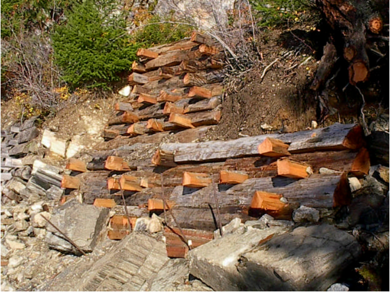
Photo 3. E-70A-5B, East Bank Trail, contingency cribbing site.
