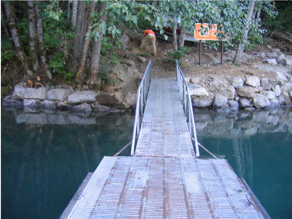
Photo 2: Buster Brown Campground after construction of rock wall in Sept. 2007.
