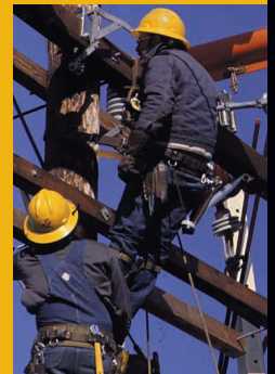
Lineworkers improving distribution system
