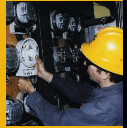
Installing new meters to add services
