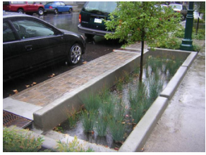
Green Stormwater Infrastructure (GSI) rain garden.
