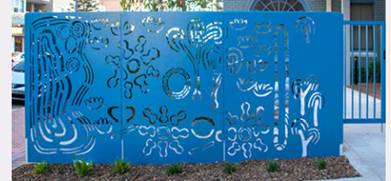
Laser cut, powder coated panels are durable and provide visually interesting panels that reflect local culture and community.
