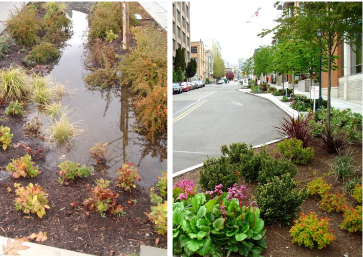
Stormwater raingarden and abundantly planted curb bulb
