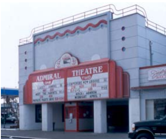
D-1: As an iconic neighborhood building, the theater exhibits several - albeit embellished - pedestrian-friendly elements. The open, visually engaging entrance from the sidewalk promotes activity in the heart of the Admiral business district.
