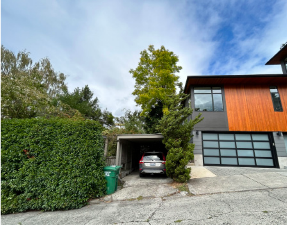
2500 MINOR AVE E- EXISTING PARKING PAD AT SE SITE
