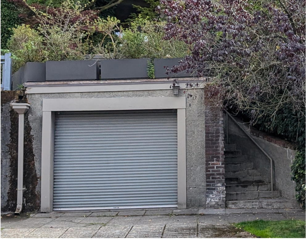
2500 MINOR AVE E - BUNKER GARAGE AT NW SITE
