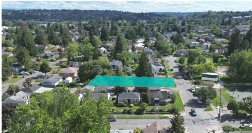
A5 ~ AERIAL LOOKING SOUTH
