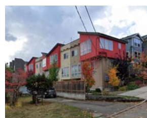
8 | 4329 S Webster St | Residential (precedent for shed roof design and transition to adjacent sites)
