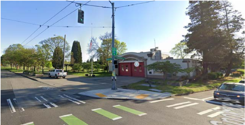
3. Seattle Fire Station 13
