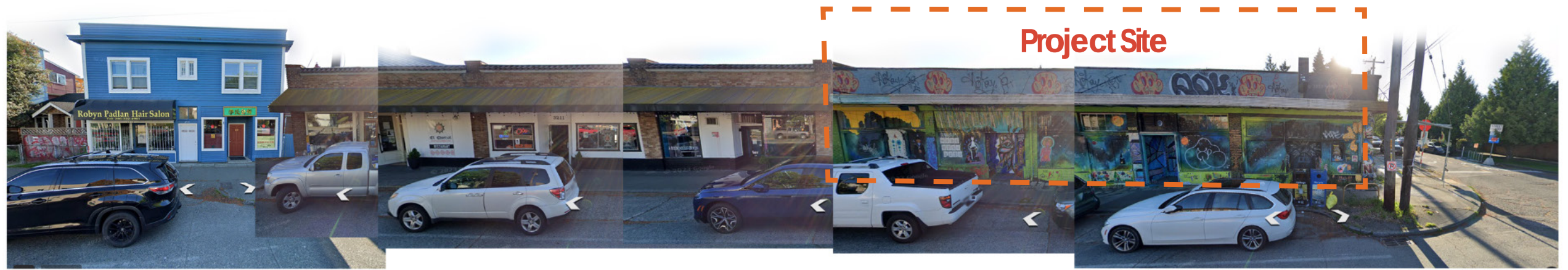
A) BEACON AVE S WEST VIEW
