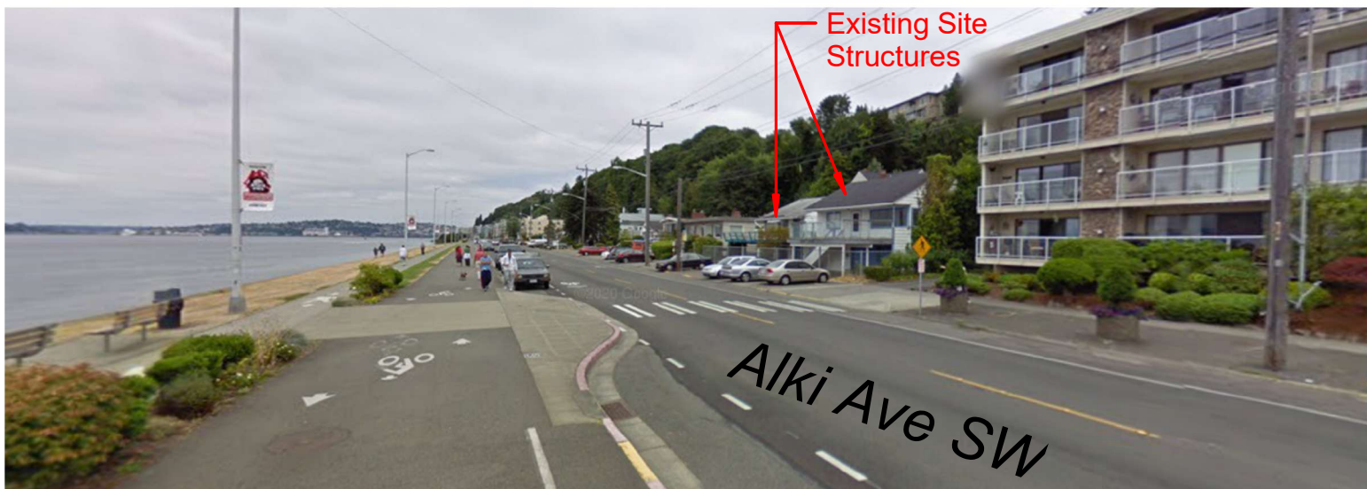
Streetview of existing neighborhood site showing different modes of access.
