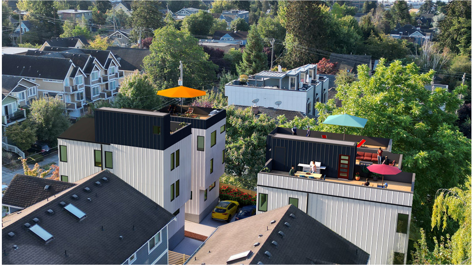
5. COURTYARD VIEW | LOOKING NORTH
