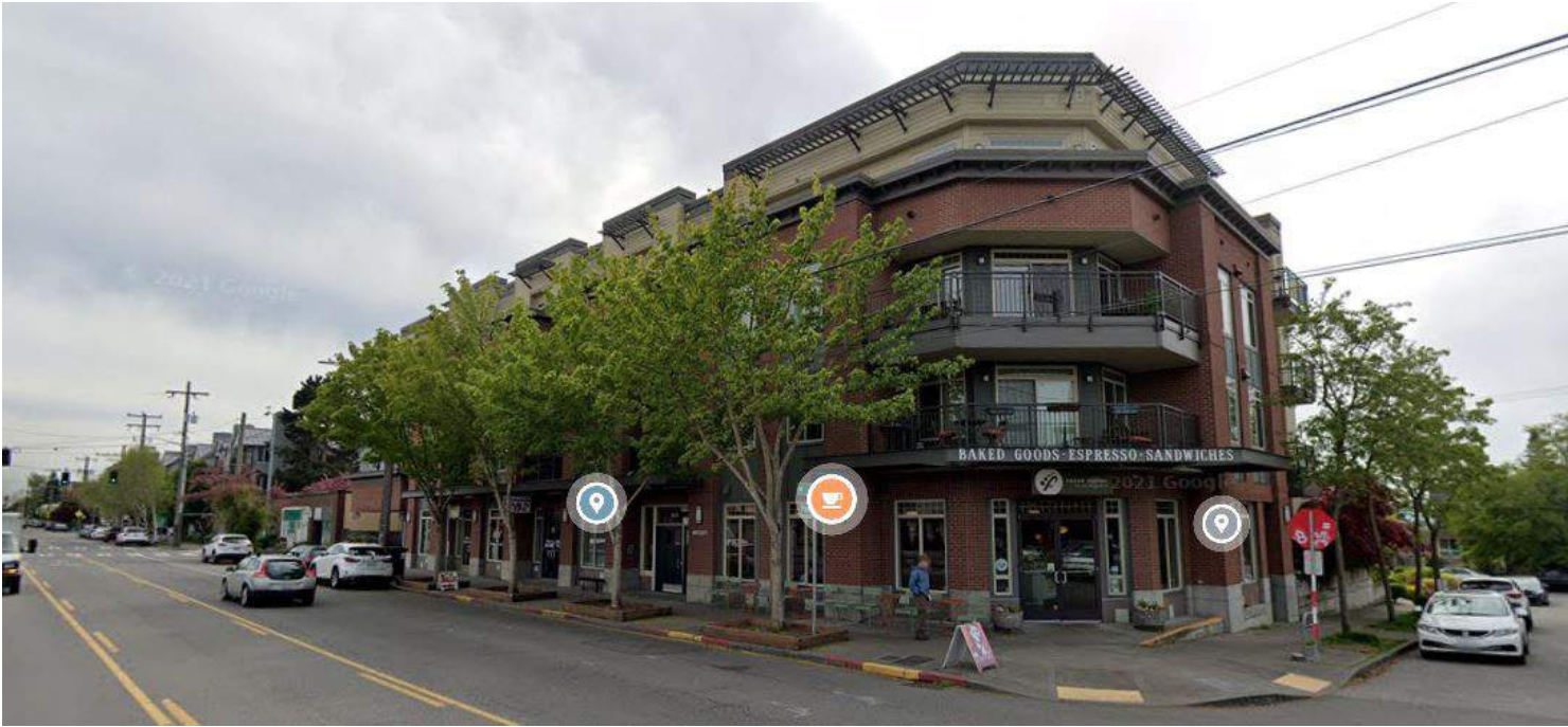
mixed-use building at 6015 Phinney Ave N with a prominent corner commercial entry condition
