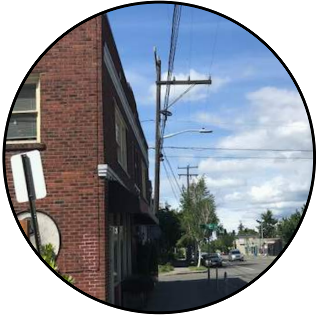
POWERLINE AT NORTHEAST CORNER
