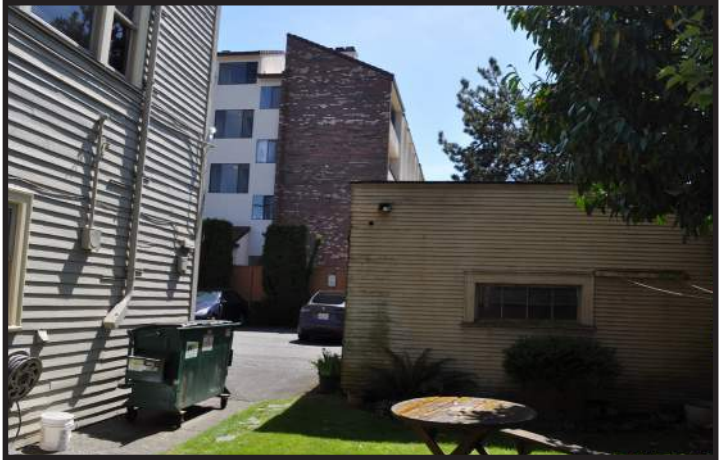
6 adjacent property line from west property line
