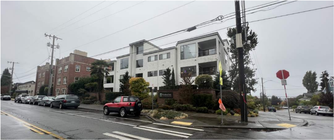
fenestration strategy @ apartment building south of project site - variations in fenestration sizes responsive to interior space function - volumes feature prominently in the overall composition
