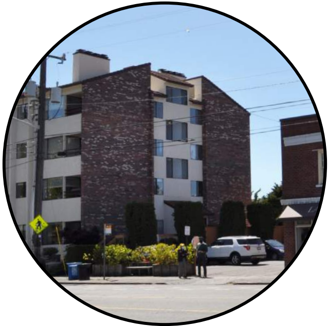
NORTH FACADE OF CONDOMINIUM BUILDING TO THE SOUTH
