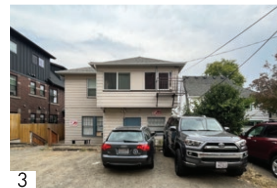
3 4753 18TH AVE NE 4753 18TH AVENUE NE | ROOMING HOUSE 2 stories rooming house located east from the project site right across the alley. Primarily uses hardie panel for exterior finishes.
