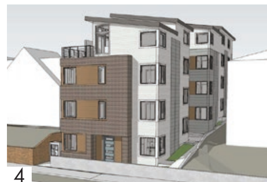
4 UW 3.0 18TH AVE 4741 18TH AVENUE NE | APARTMENT 2 identical apartment buildings that each have 4 stories, each with a private deck on top floor. Currently under construction. Primarily uses hardie panel, brick and wood for exterior finishes.
