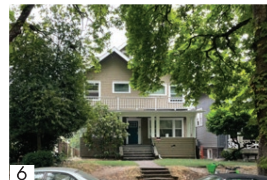
6 4738 17TH AVE NE 4738 17TH AVENUE NE | ROOMING HOUSE 2 stories rooming house located south, right next to the project site. Primarily used hardie panel for exterior finishes.
