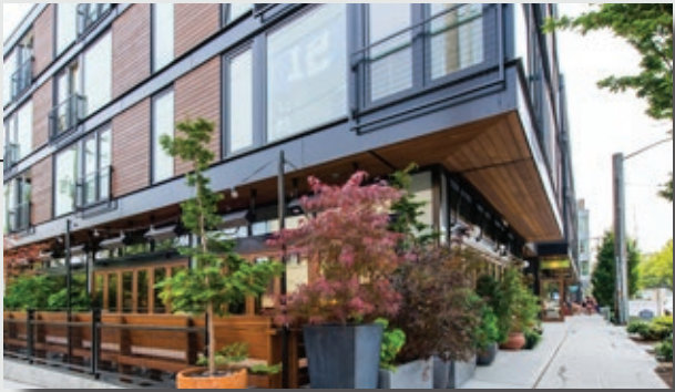
Cantilevered weather protection
