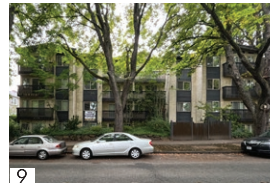
9 TAMARAC APARTMENT 4733 17TH AVENUE NE | APARTMENT 4 stories apartment building located south west from the project site. Primarily uses concrete and wood for exterior finishes
