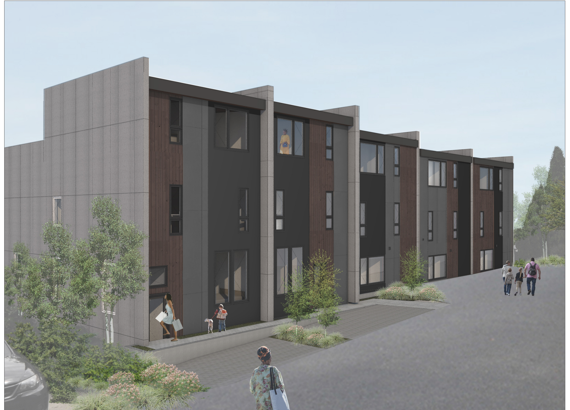
3. Rear View looking Southeast
