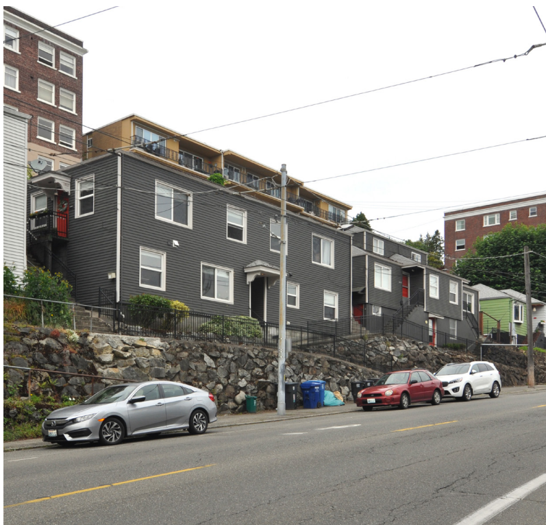
2 View facing Northwest looking at site
