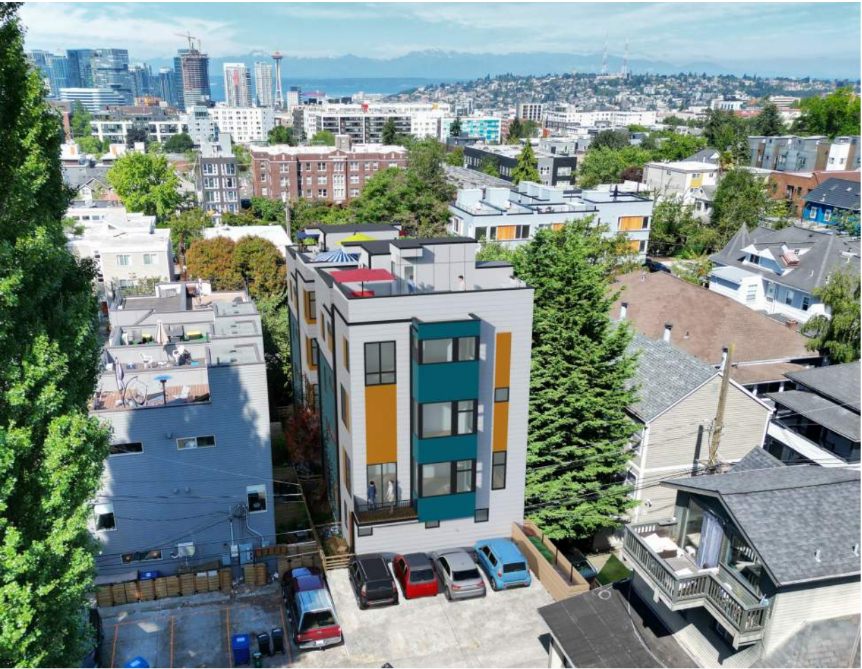
2. AERIAL VIEW REAR FACADE
