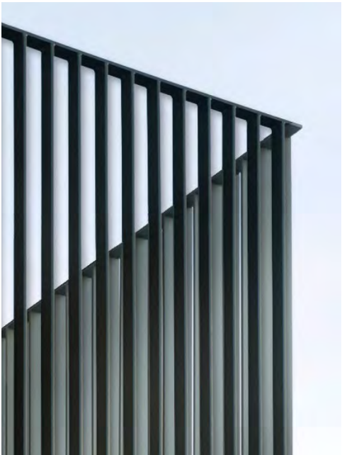
8 Steel Flat Bar Guards Powder Coated Black 1 1/2" x 1/2"
