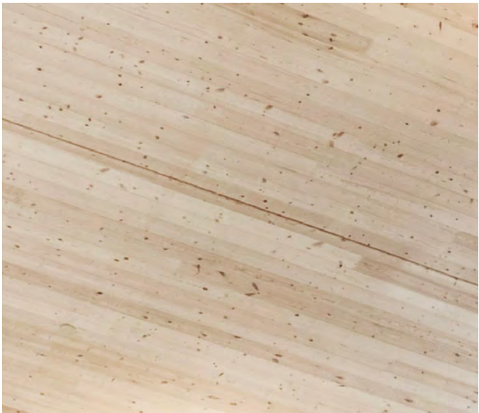
2 Exposed CLT Ceilings Interior & Exterior 3-ply (3 1/2") at canopies / 5-ply (5 1/2") at upper levels
