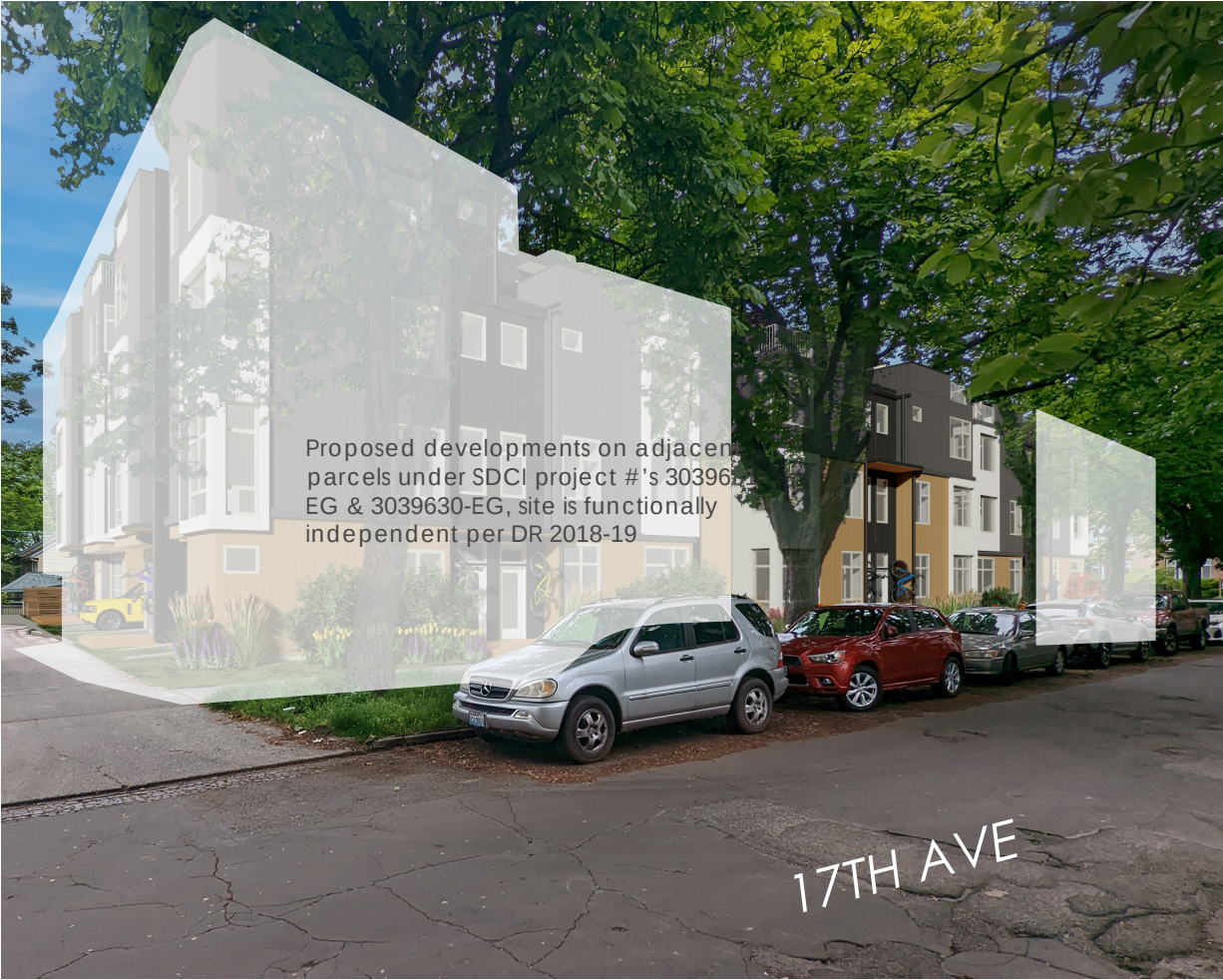
1. APPROACH FROM SOUTHEAST ACROSS 17TH AVE
