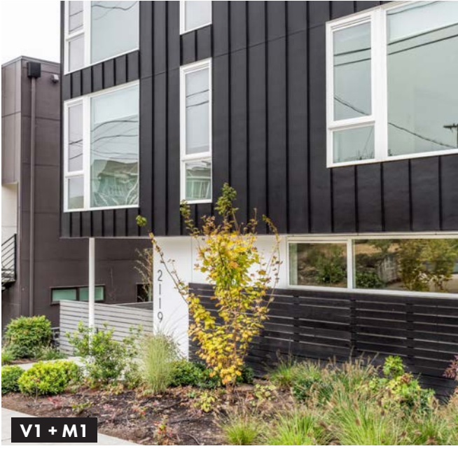
Plygem Windows Vinyl (Window Frames) + Steel Columns
