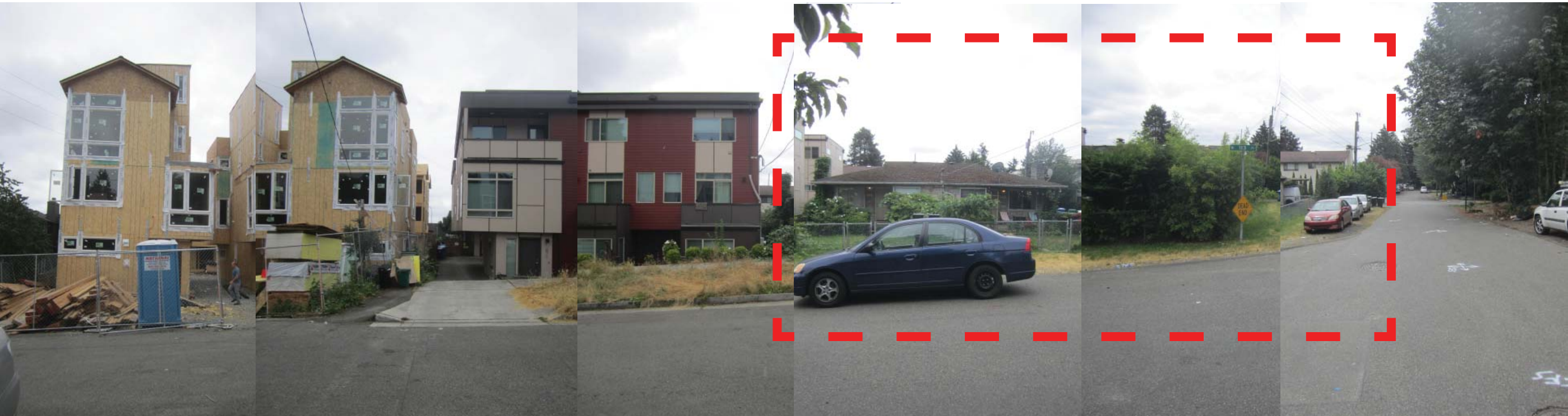
N 113TH STREET LOOKING SOUTH
