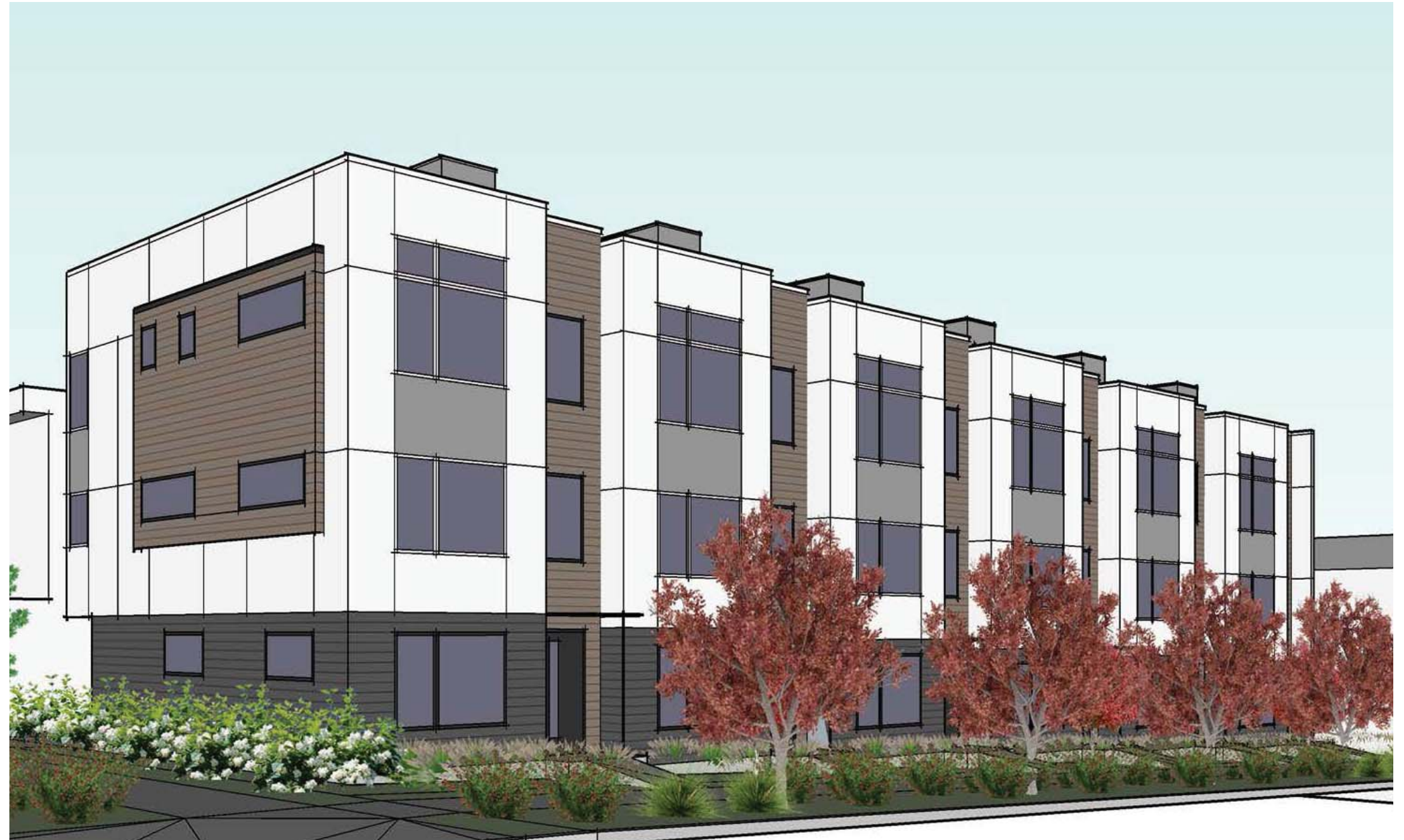
STREET CORNER AT NORTHWEST
