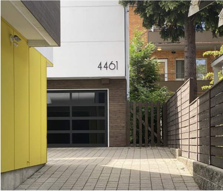
4461 MIDVALE AVE N (8.8) VISIBLE GARAGE FROM STREET.
