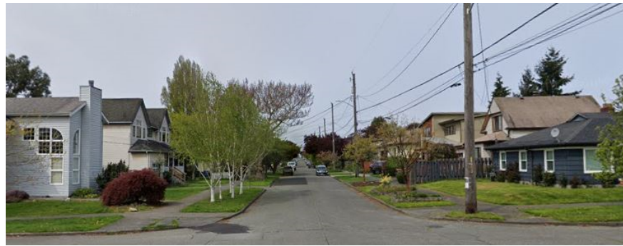
LOOKING WEST ON NW 59 TH STREET
