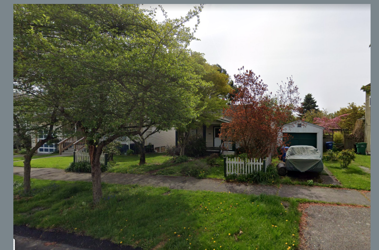
EXISTING SITE PHOTOS
