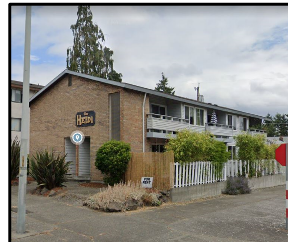
5 6201 14 th Avenue NW Existing Small Apartments
