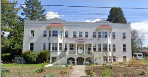
Existing structure across street.
