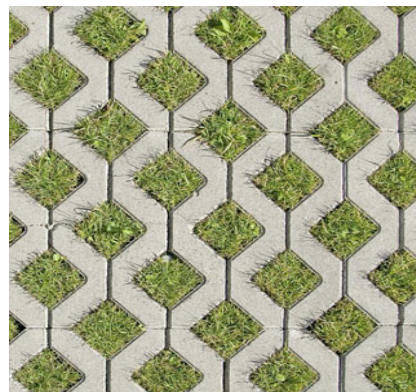
Permeable grasscrete pavers
