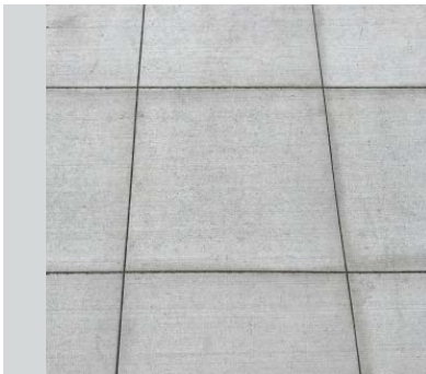
CONCRETE 2'X 2' SIDEWALK, NO SHINERS
