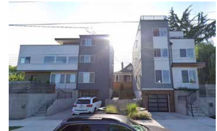
4. Multifamily Townhouse 6511 44th Ave S
