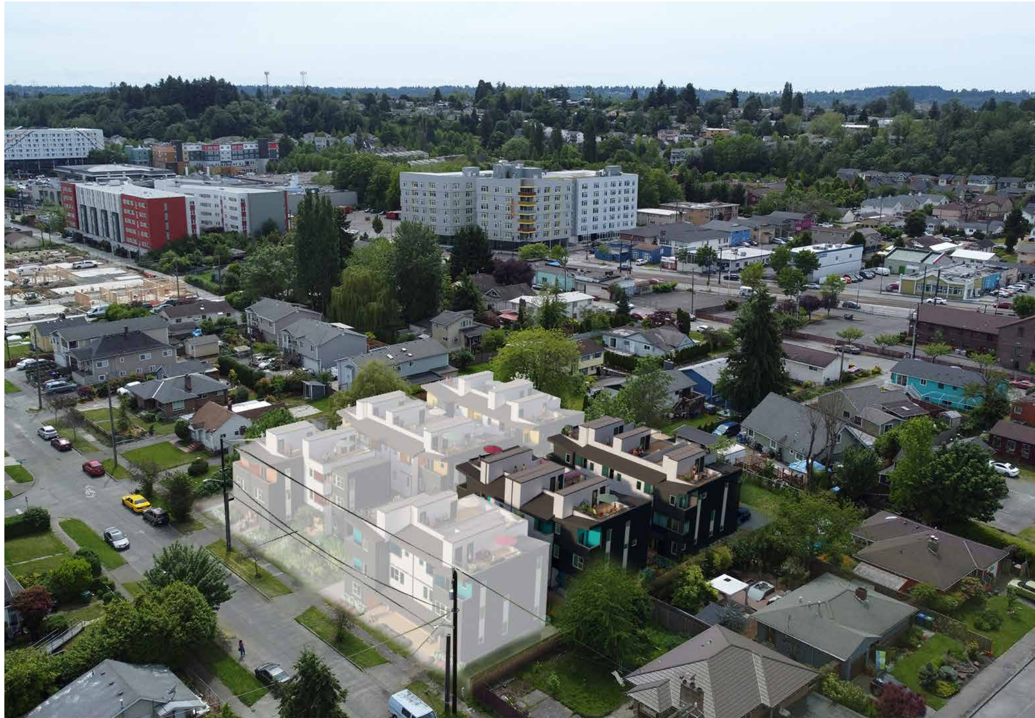
5. AERIAL VIEW FROM CORNER OF S HOLLY ST AND 42ND AVE S
