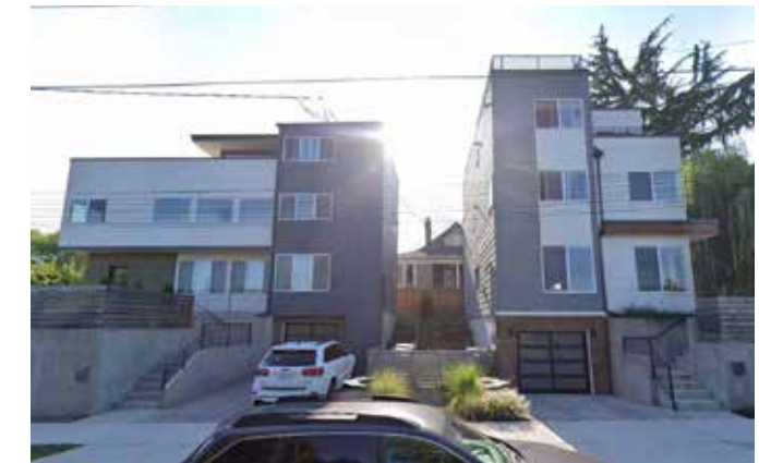
4. Multifamily Townhouse 6511 44th Ave S
