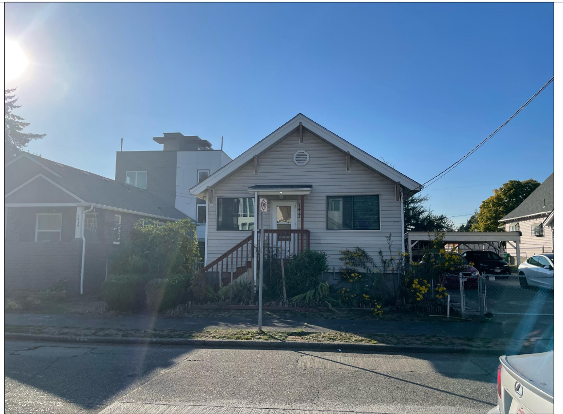
EAST FACADE OF EXISTING HOUSE FROM ALAMO ST S
