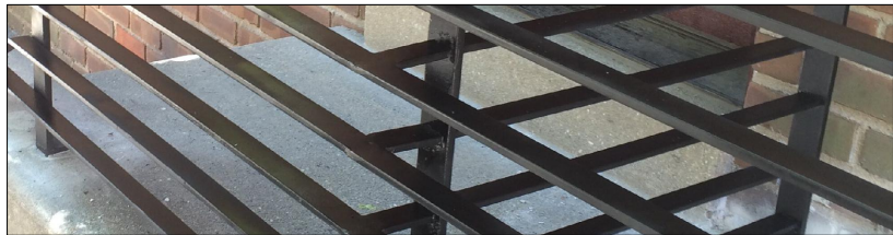
BLACK PAINTED STEEL RAILINGS AND DETAILS, \frac{3}{8} " x 2" FLAT BAR, THROUGHOUT, RAL#9005
