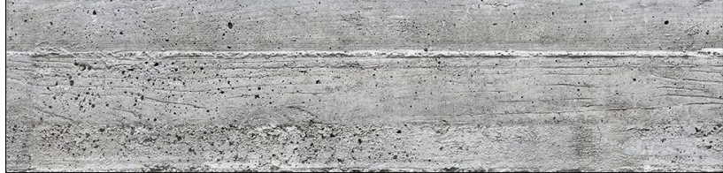
BOARD FORMED CONCRETE
