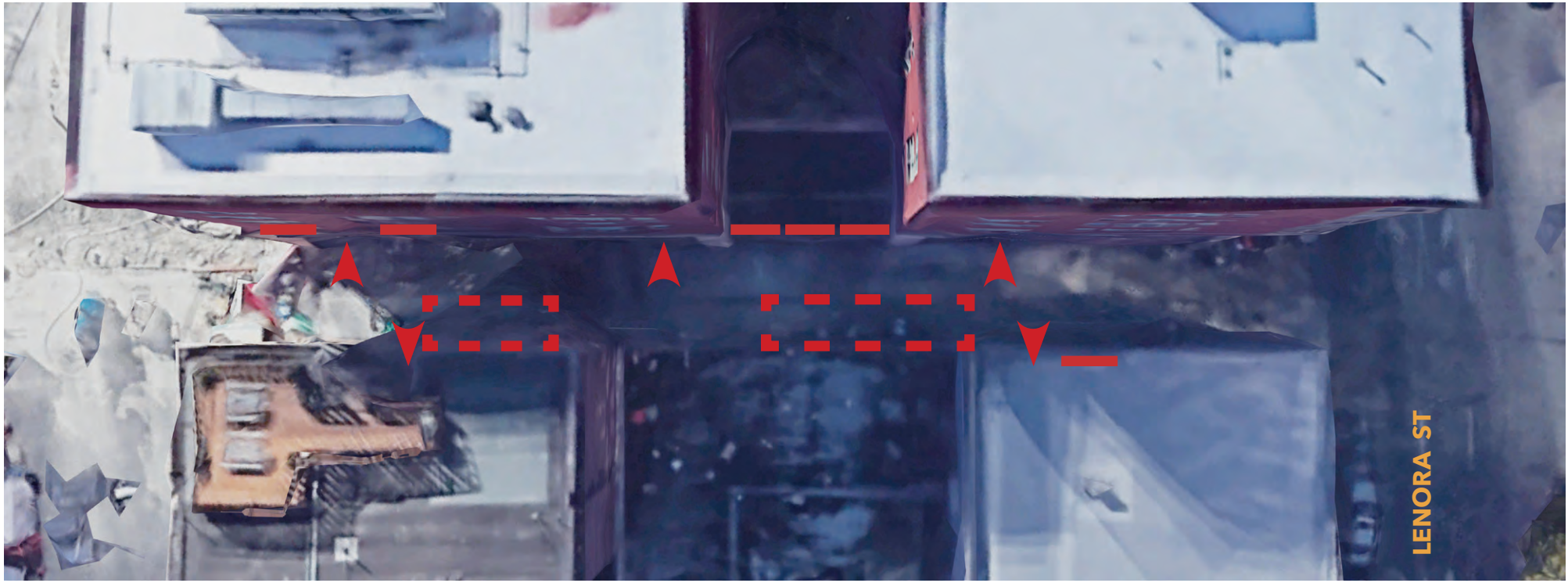
EXISTING ALLEY CONDITION
