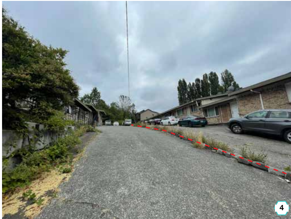
• ON-SITE LOOKING EAST
