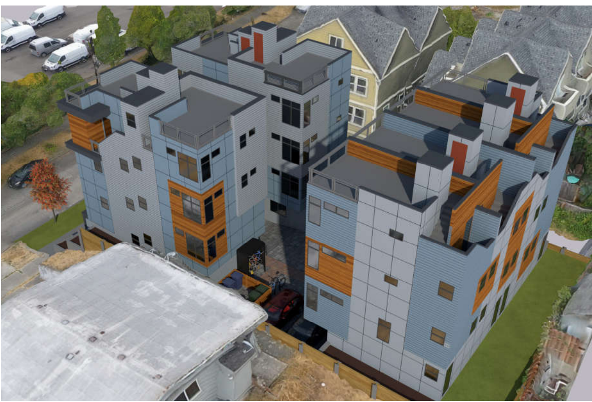
AERIAL VIEW LOOKING NORTHWEST
