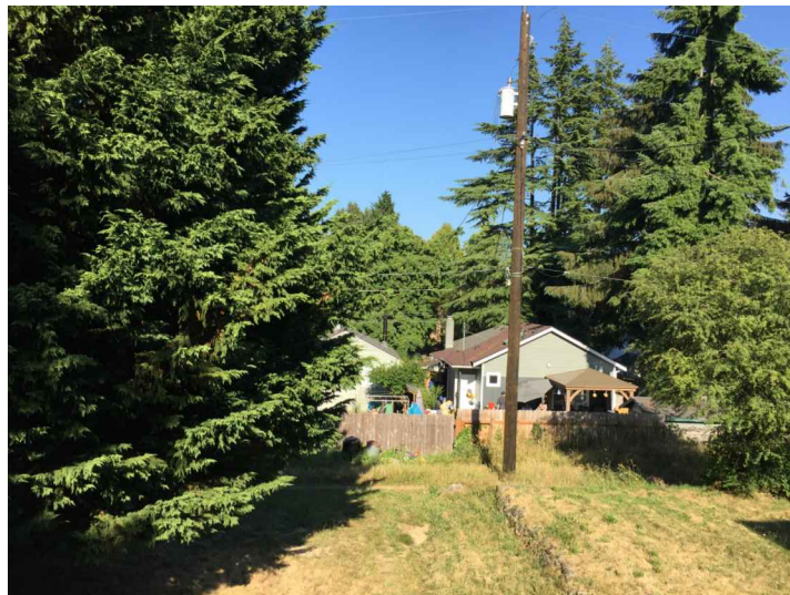
POWER LINE AT ALLEY
