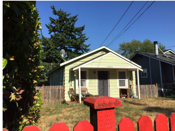
EXISTING ONE STORY #10034 SINGLE FAMILY
