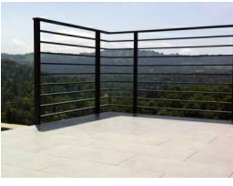
Open Steel railing
