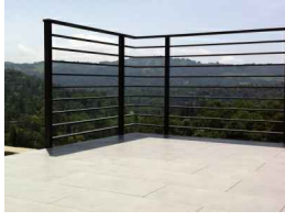
Open Steel railing
