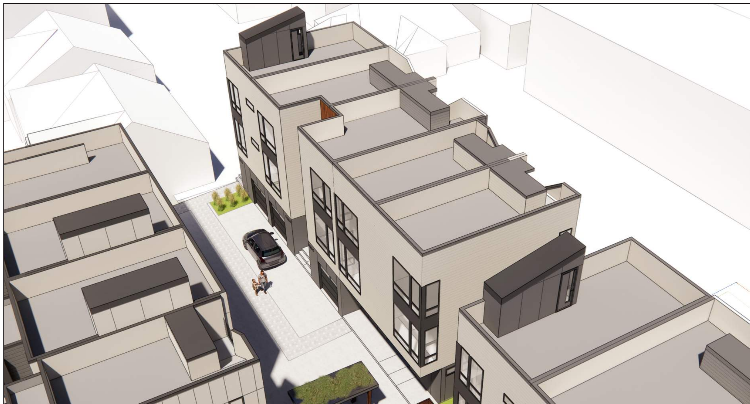
LOOKING NORTHEAST AT REAR OF BUILDING
