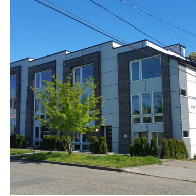
7. 5912 Fauntleroy Way SW 3 Stories Townhouse 5 Units
