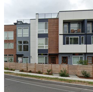
4. 5913 California Ave SW 3 stories Townhouse 3 units
