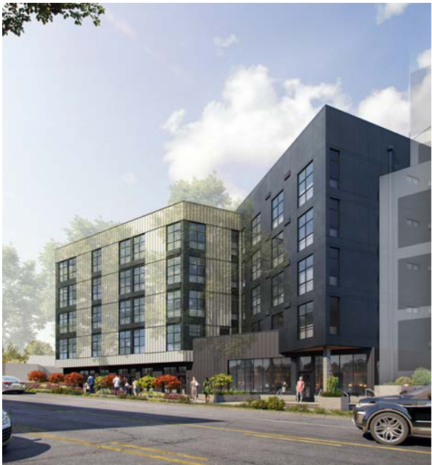
5231 Rainier Ave S (Under Construction)
