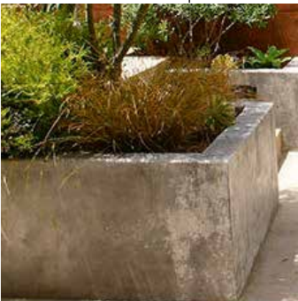
Planter, Cast-in-place Concrete Concrete planter at seat height.
