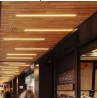
Recessed Linear Lighting in Wood Soffit A canopy provides weather protection and lighting.
