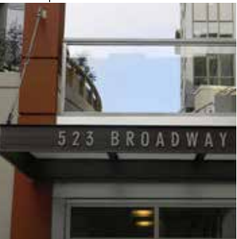
Canopy Signage Signage at canopy edge emphasizes corner entry and lobby.
