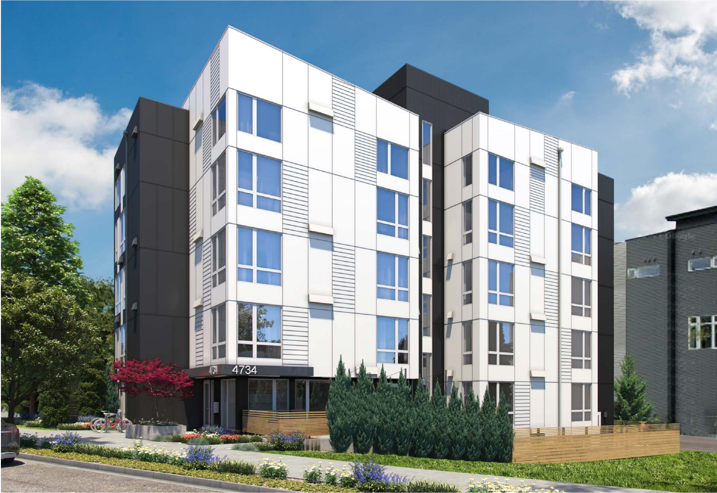
View from Southwest Corner
